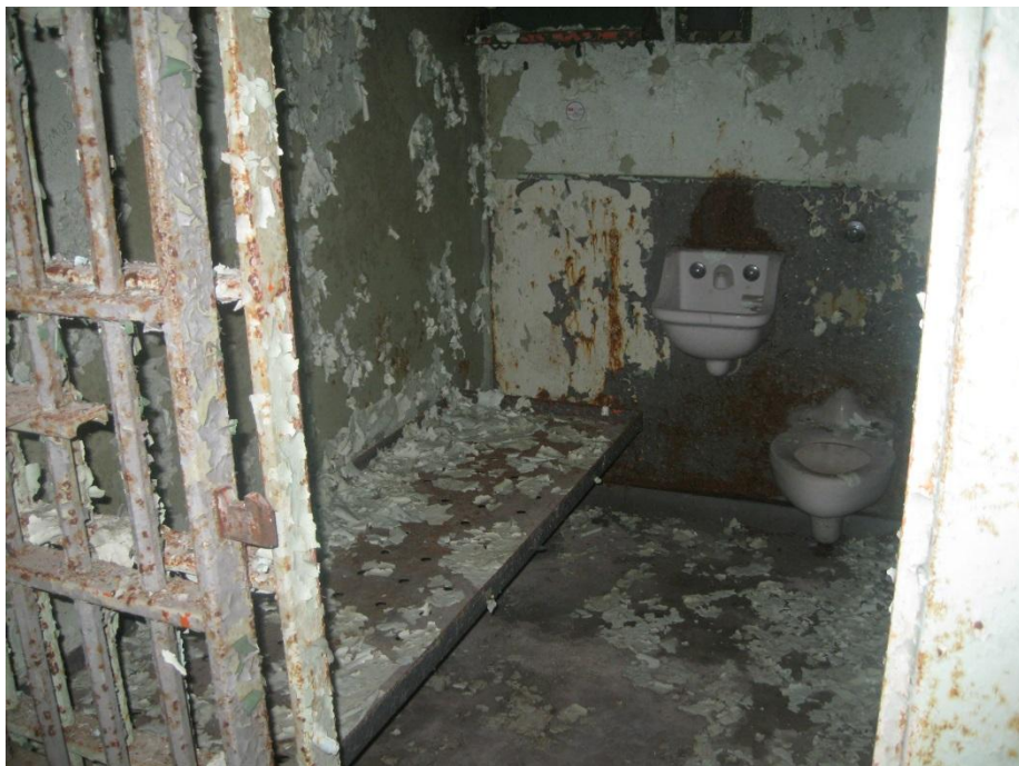
Photo J-16 – Chipping Paint and Rust at Steel in Cell Block
