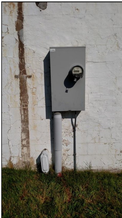
Photo 4 – Pump house Electrical Panel
