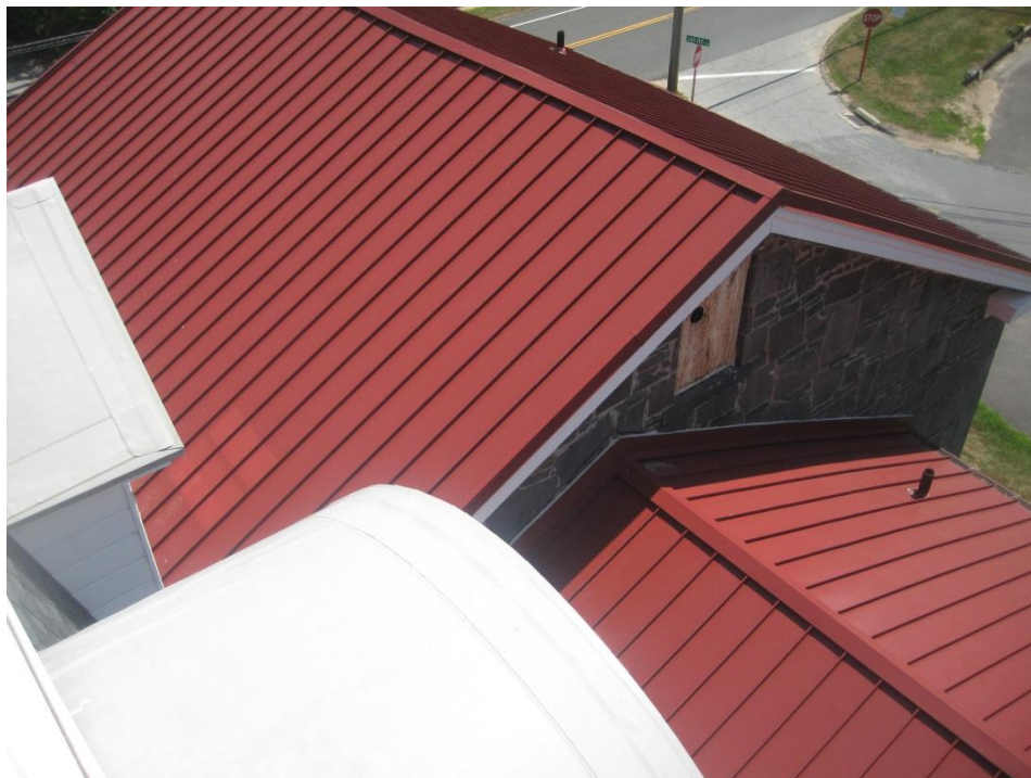
Photo J-2 – Standing Seam Metal Roof Over Cell Block
