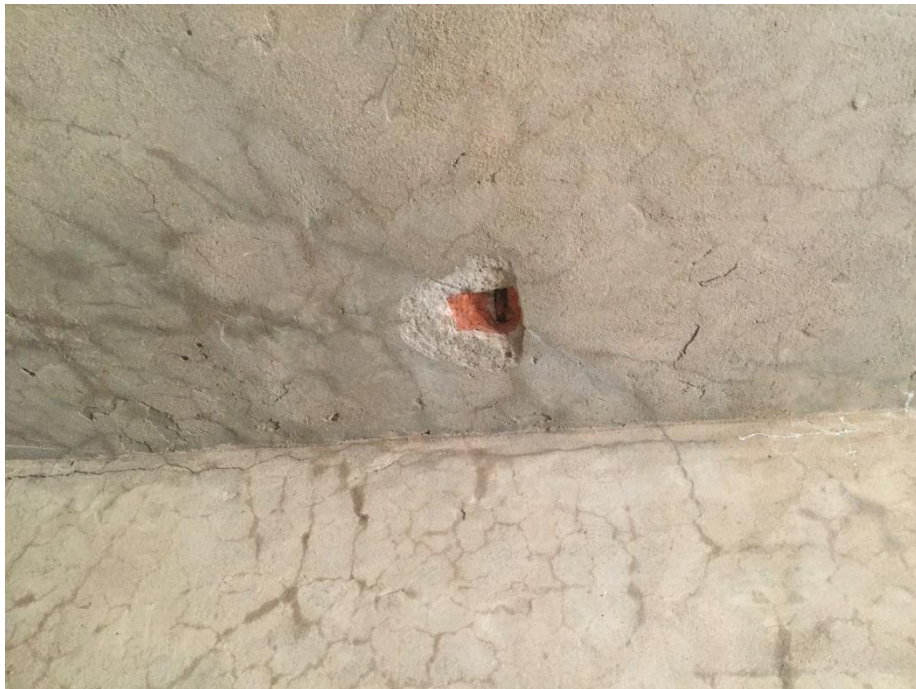
Photo P-5 – Apparent Clay Masonry at Pump House Roof
