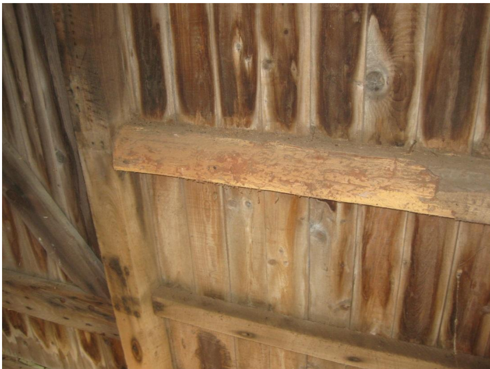
Photo C-5 – Modifications and Damage to Wall Framing at Corn House
