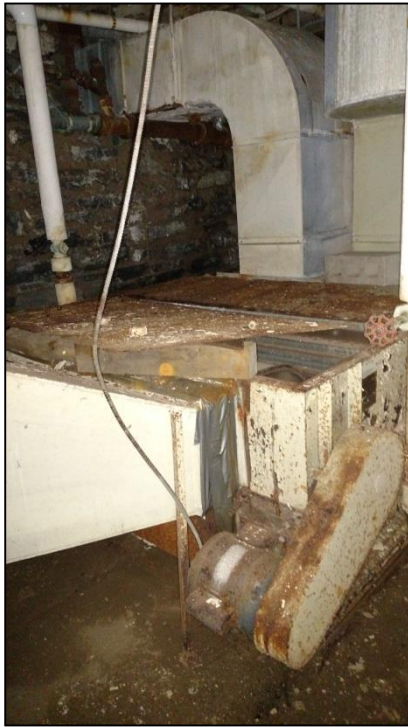
Photo 5 – Jailhouse Building Air Handling Unit
