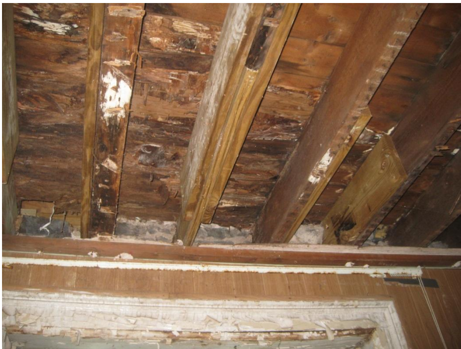
Photo J-8 – Reinforced Floor Joists
