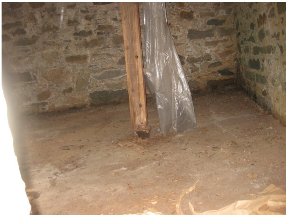
Photo C-3 – Deteriorated Post at Shoring
