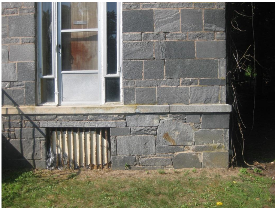
Photo J-12 – Mortar Degradation at Exterior Walls of Admin Building
