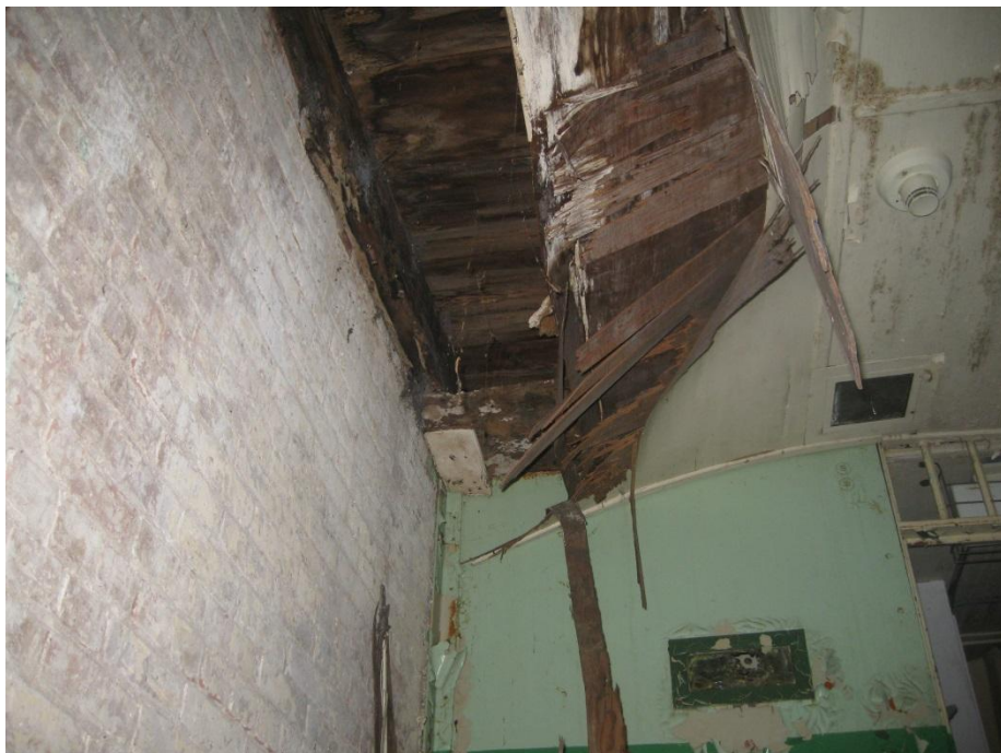
Photo J-18 – Ceiling Damage at Cell Block
