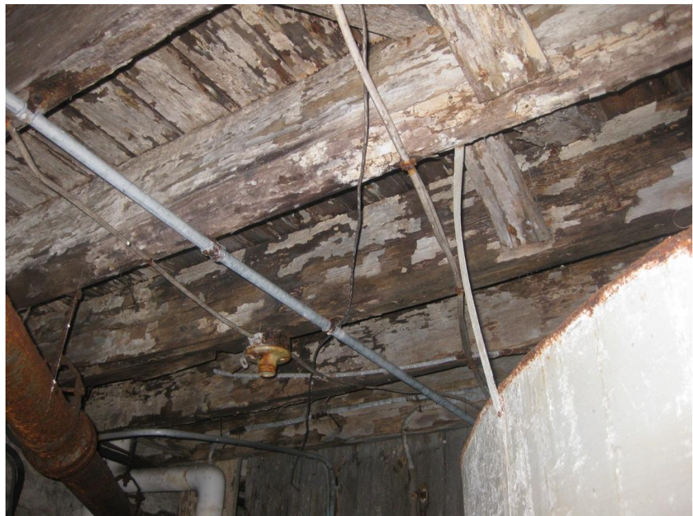
Photo J-6 – Deteriorated Floor Elements at Southwest Corner
