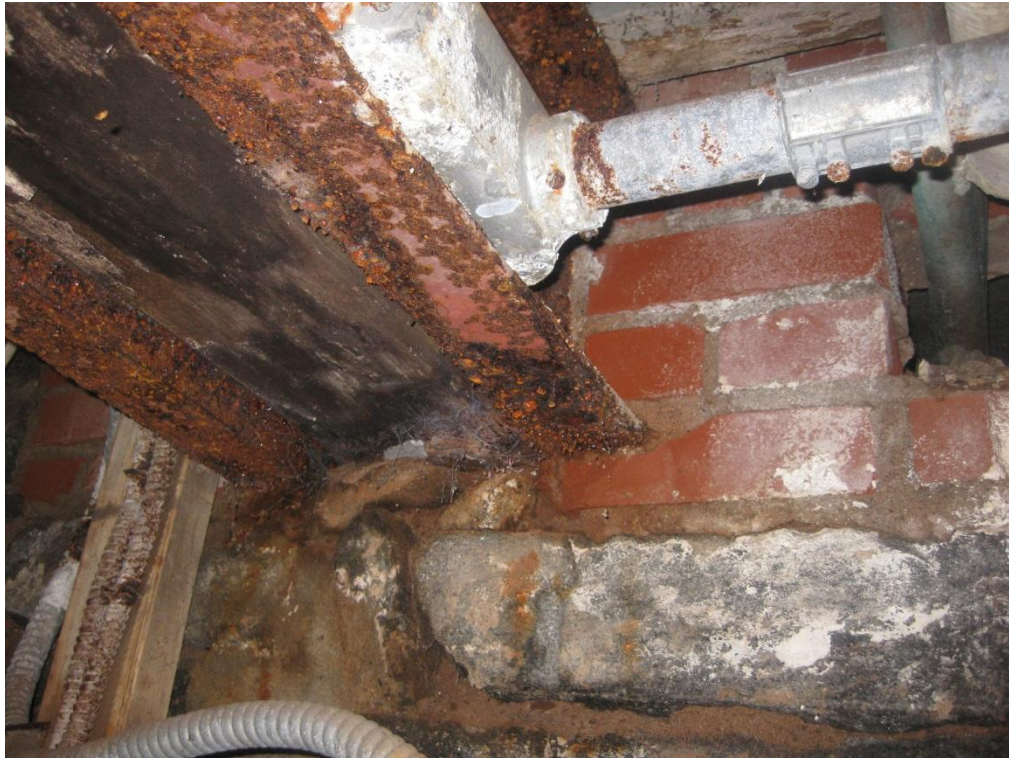
Photo J-5 – Water Infiltration at Channel Reinforcing
