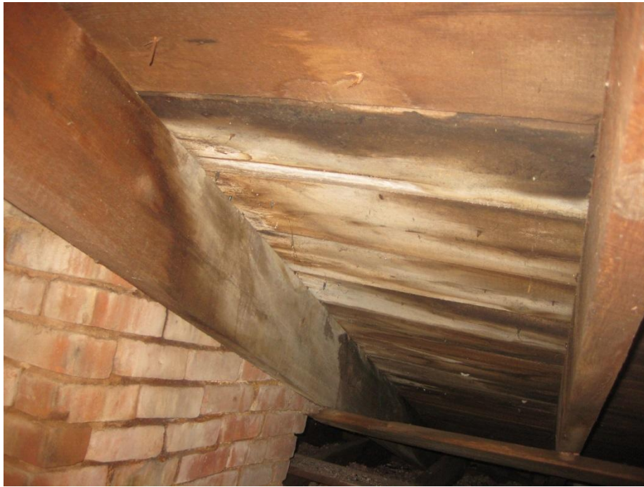
Photo J-11 – Signs of Water Infiltration at Admin Roof Framing
