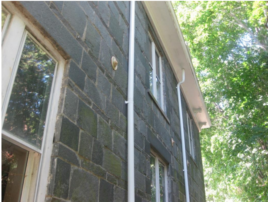
Photo J-13 – Masonry Anchors and Cornice at North Wall
