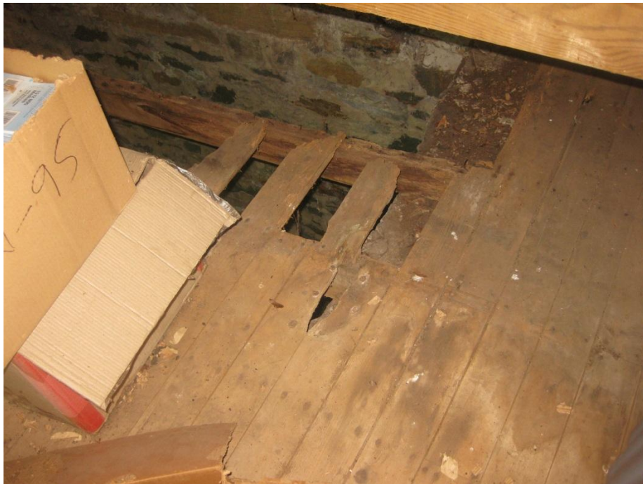
Photo C-4 – Deteriorated Floor Boards at Corn House
