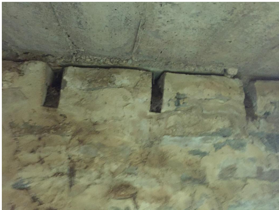
Photo R-5 – Bearing Pockets at Wall of Root Cellar
