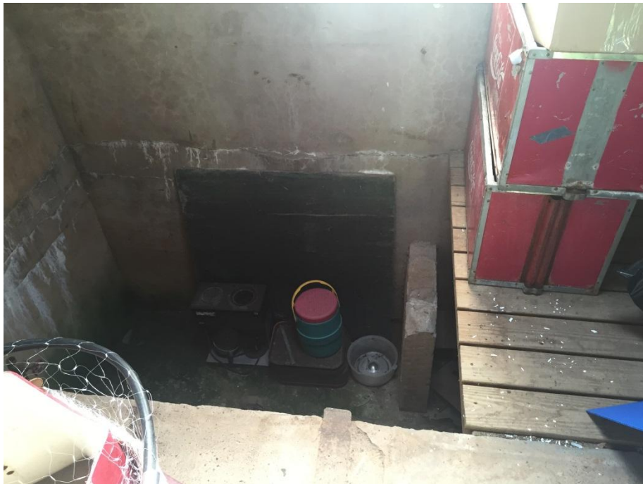
Photo P-4 – Cracks and Efflorescence at Pit at Pump House
