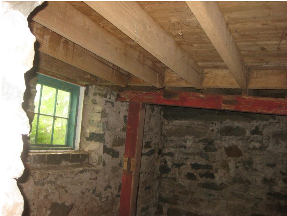
Photo C-2 – Shoring Not in Contact With Floor Framing
