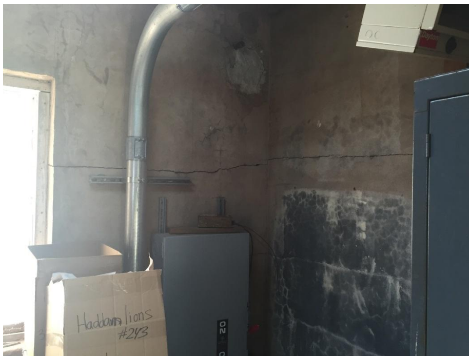
Photo P-2 – Large Horizontal Crack at Interior of Pump House Wall
