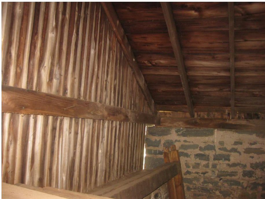
Photo S-4 – Gaps at Wall Interfaces
