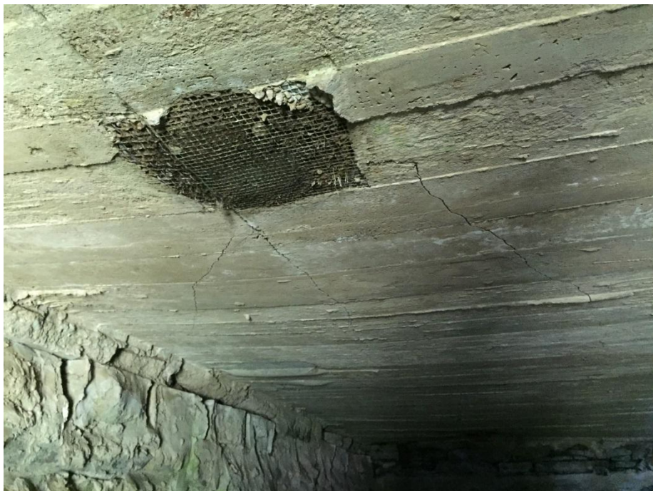
Photo R-3 – Cracks at Roof Slab at Infill at Root Cellar
