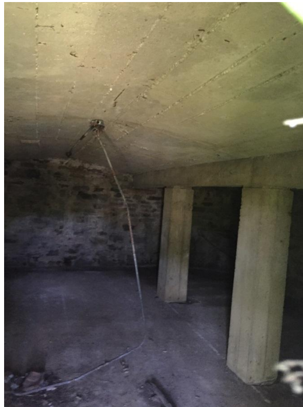
Photo R-4 – Concrete Arches and Columns at Root Cellar
