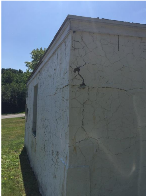
Photo P-3 – Cracked Walls at NW Corner of Pump House
