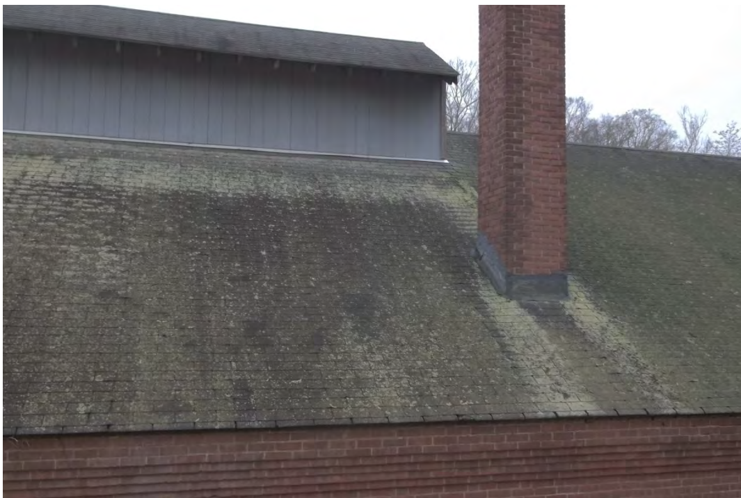
Example of asbestos-containing roof flashing materials/base flashing
