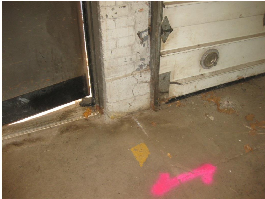
Photo A-13 – Stepped and vertical cracks at interior face of exterior wall
