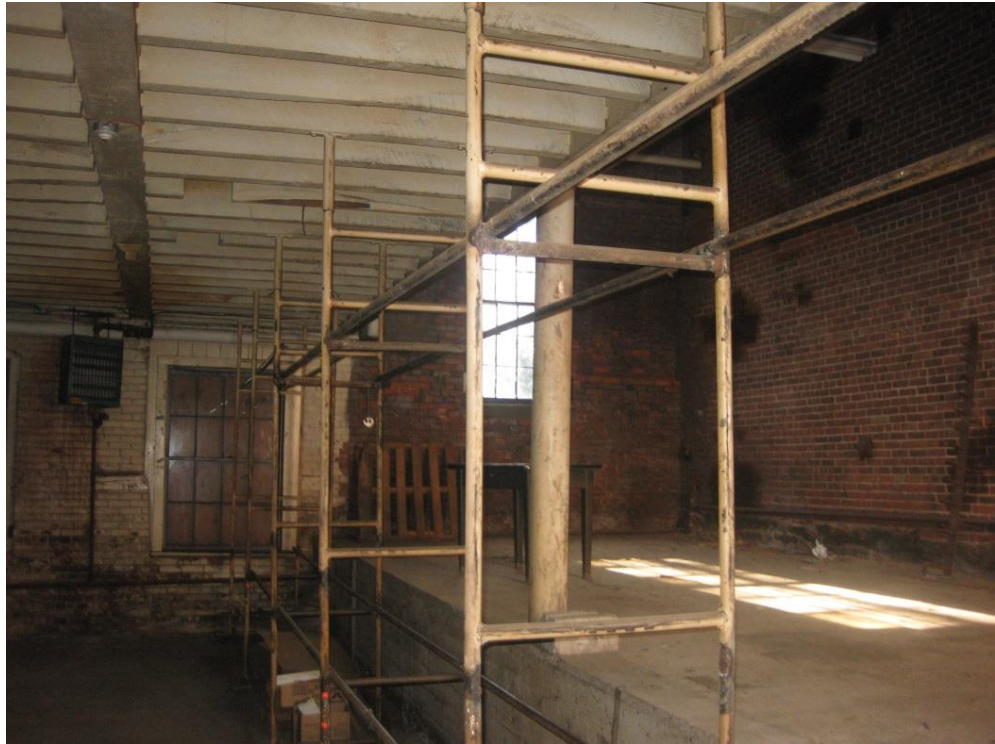
Photo B-9 – Retaining wall, framing and shoring at east end of Building B
