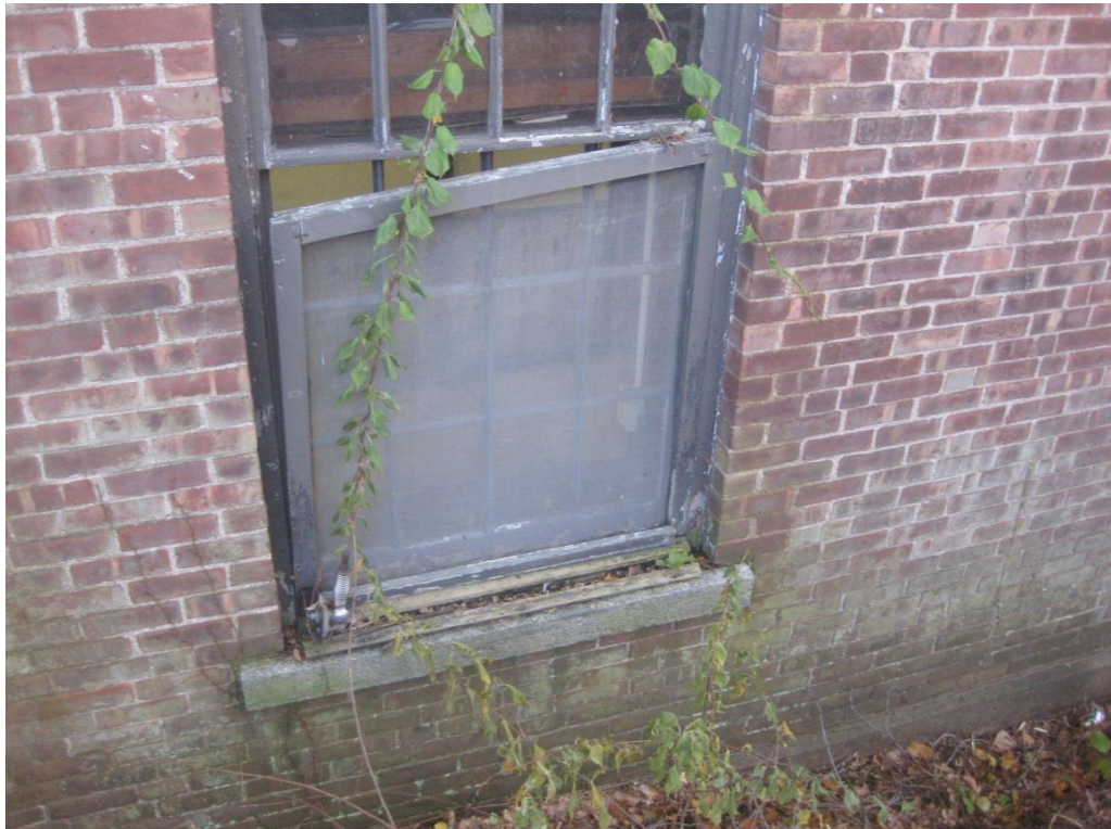
Photo A-6 – Deteriorated exterior window frame
