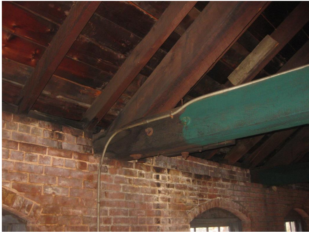
Photo B-17 – Deteriorated and weathered wood truss at wall bearing (east side)
