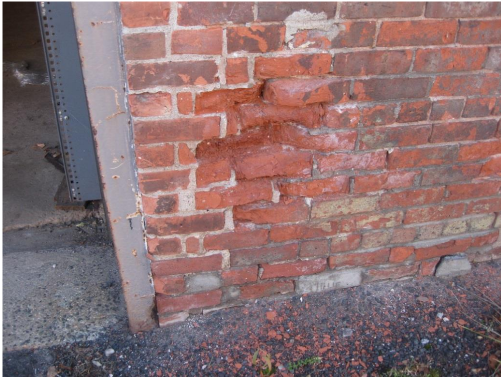
Photo B-7 – Brick damage on exterior brick wall due to impact
