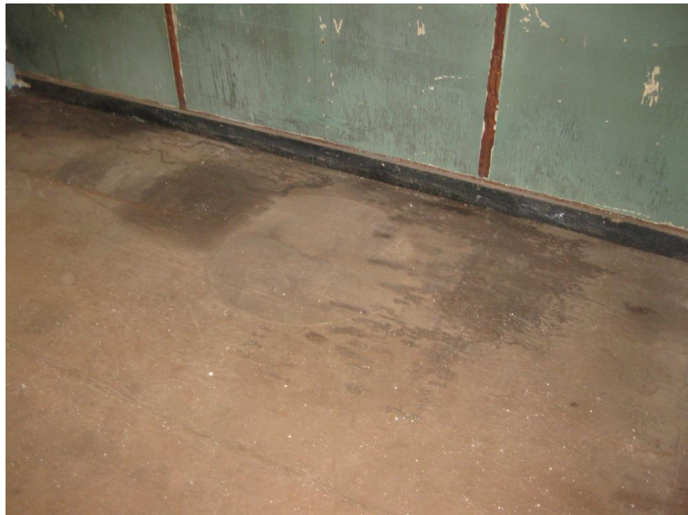
Photo A-12 – Weathered and water damaged subflooring
