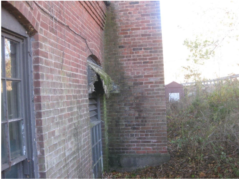
Photo A-3 – Deteriorated louver cover
