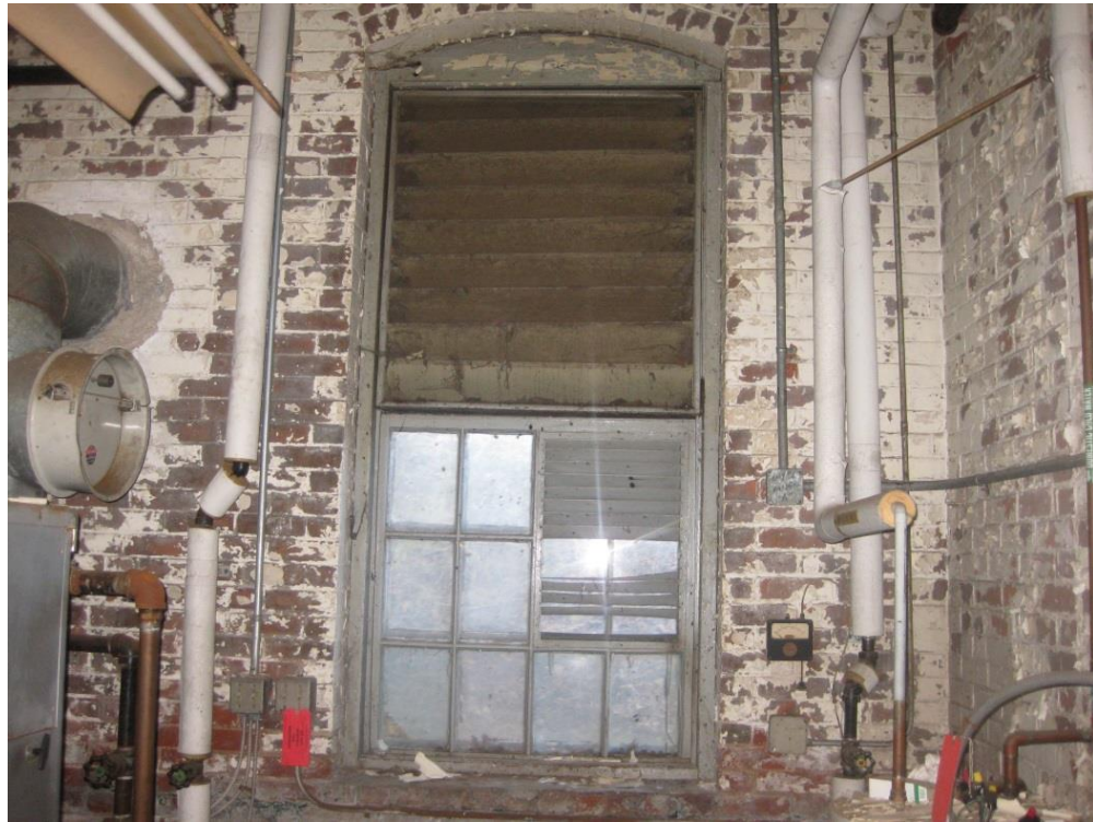
Photo A-11 – Chipped paint and deteriorated mortar at interior walls
