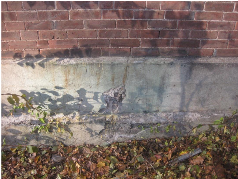
Photo A-1 – Diagonal crack and concrete spalling at foundation wall
