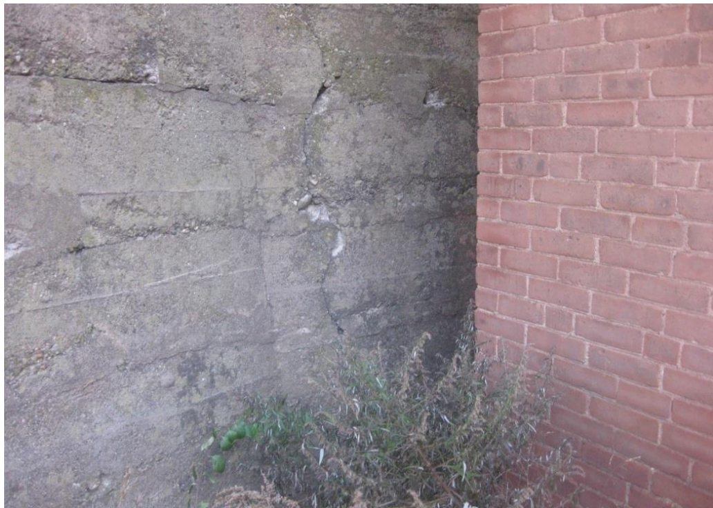
Photo A-8 – Deterioration at retaining wall parallel to rear wall of Building A
