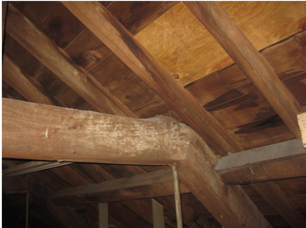
Photo B-18 – Deteriorated and weathered wooden truss (west side)
