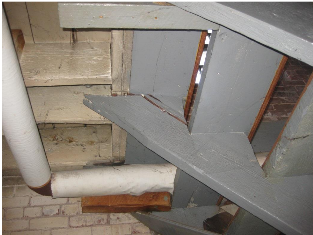
Photo B-12 – Wood stringer failure at mezzanine stair
