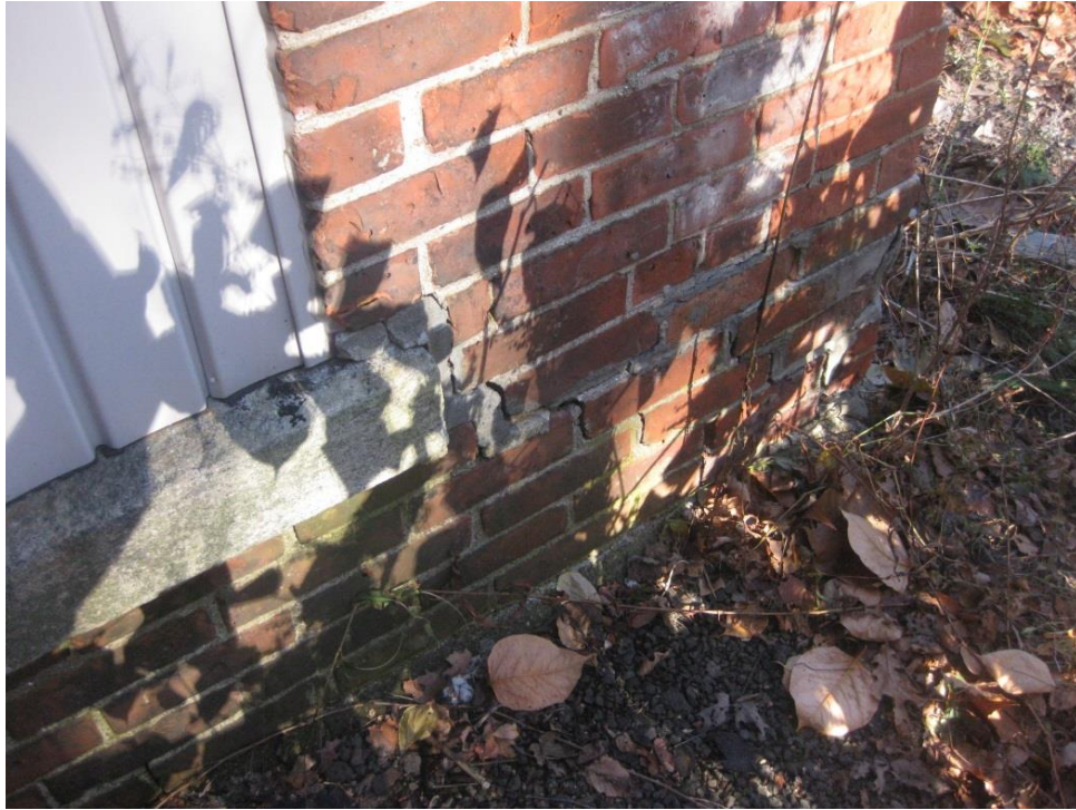
Photo B-1 – Stepped crack along mortar joint at SE corner of Building B
