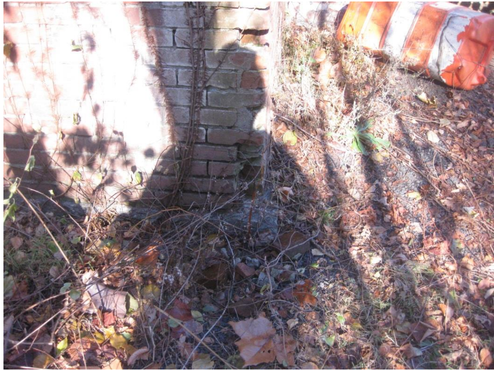
Photo B-5 – Disintegrated mortar and spalling at SE corner of Building B
