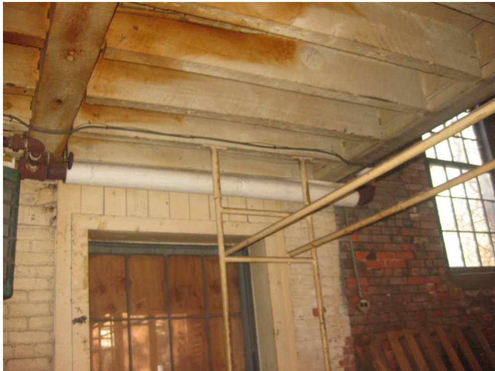
Photo B-10 –Moisture stains on wood beams at mezzanine
