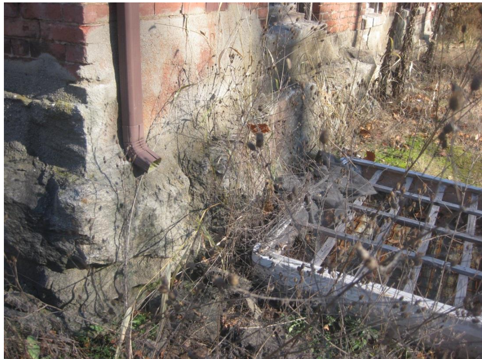
Photo B-6 – Section of exterior wall founded on rock outcropping
