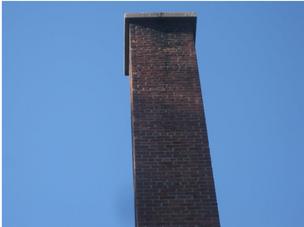
Photo B-3 – Vertical crack at the chimney of Building
