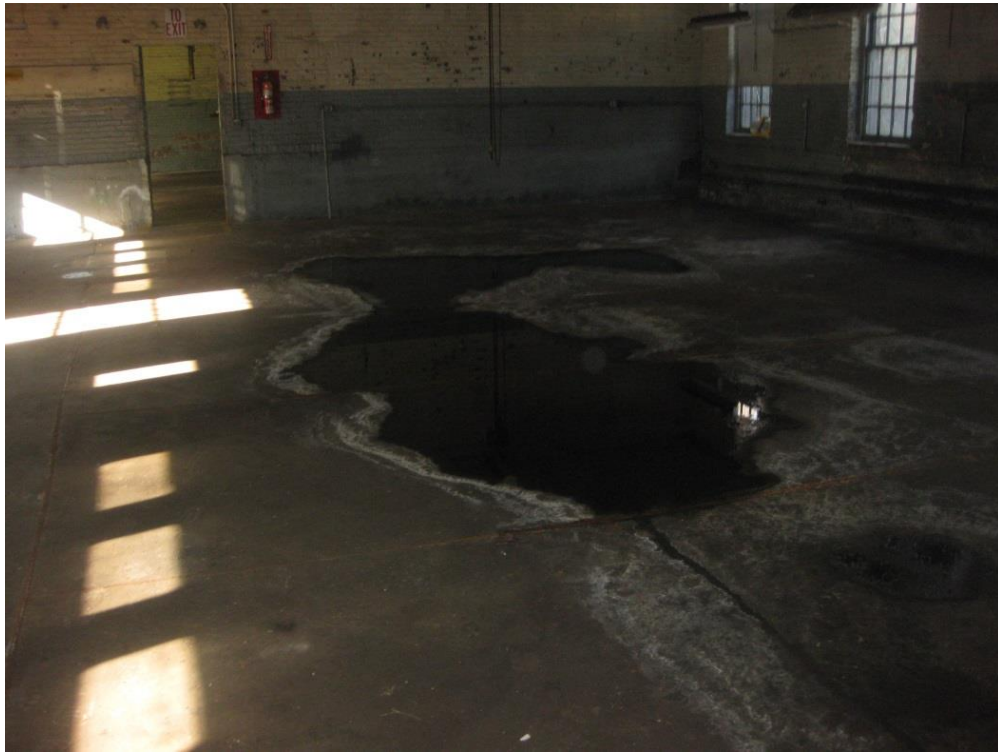
Photo A-15 – Ponding water at concrete slab sloped to center
