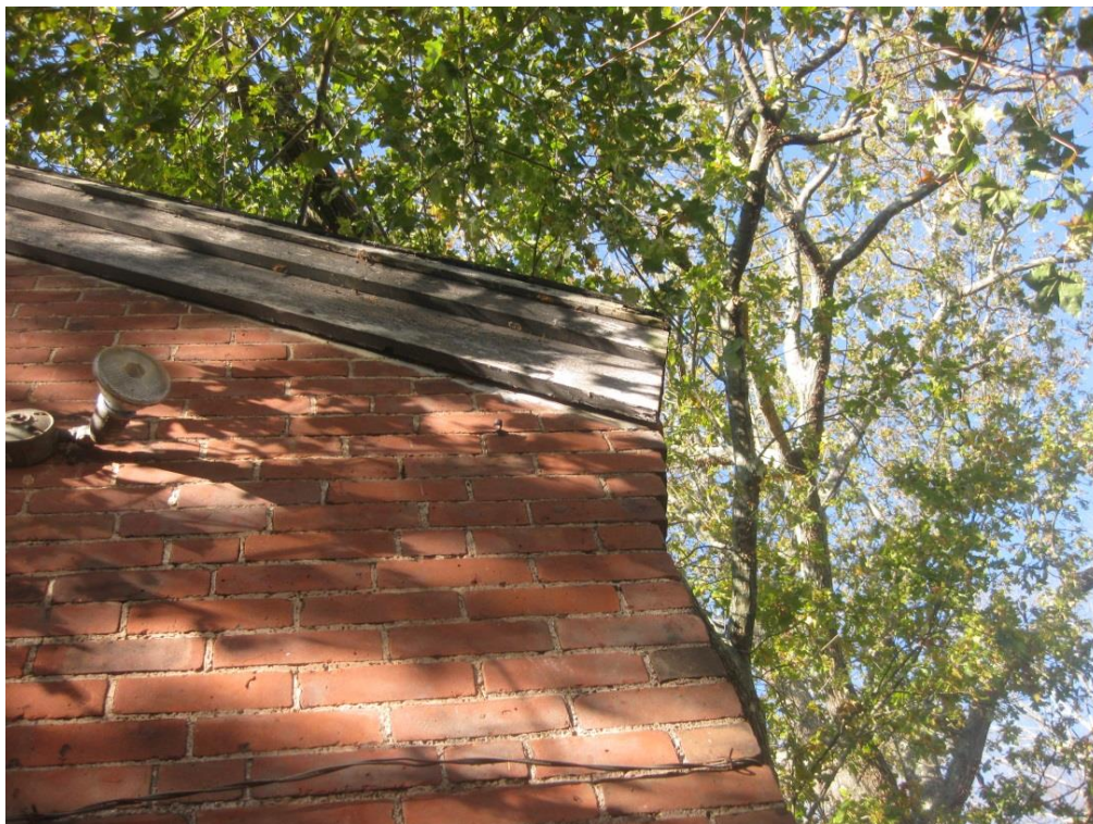
Photo A-2 – Dry and deteriorated wood fascia
