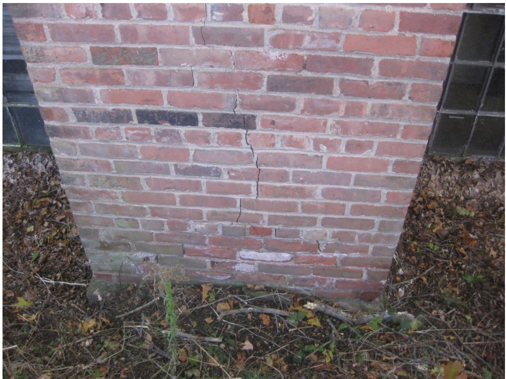
Photo A-4 – Vertical Crack along Chimney
