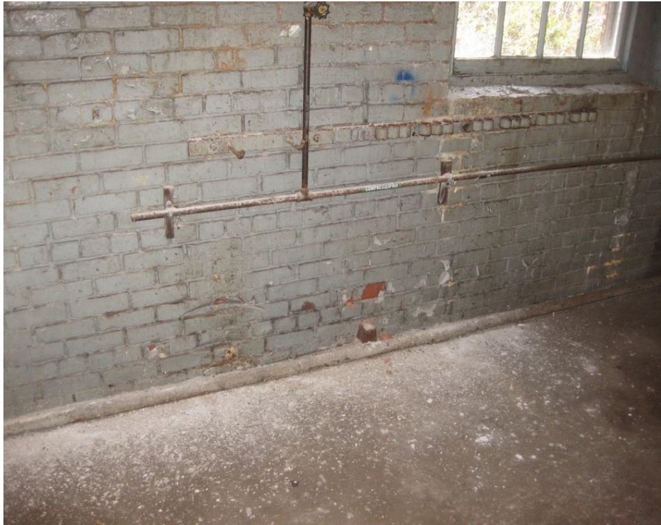
Photo B-15 – Disintegrated mortar at inside face of exterior wall
