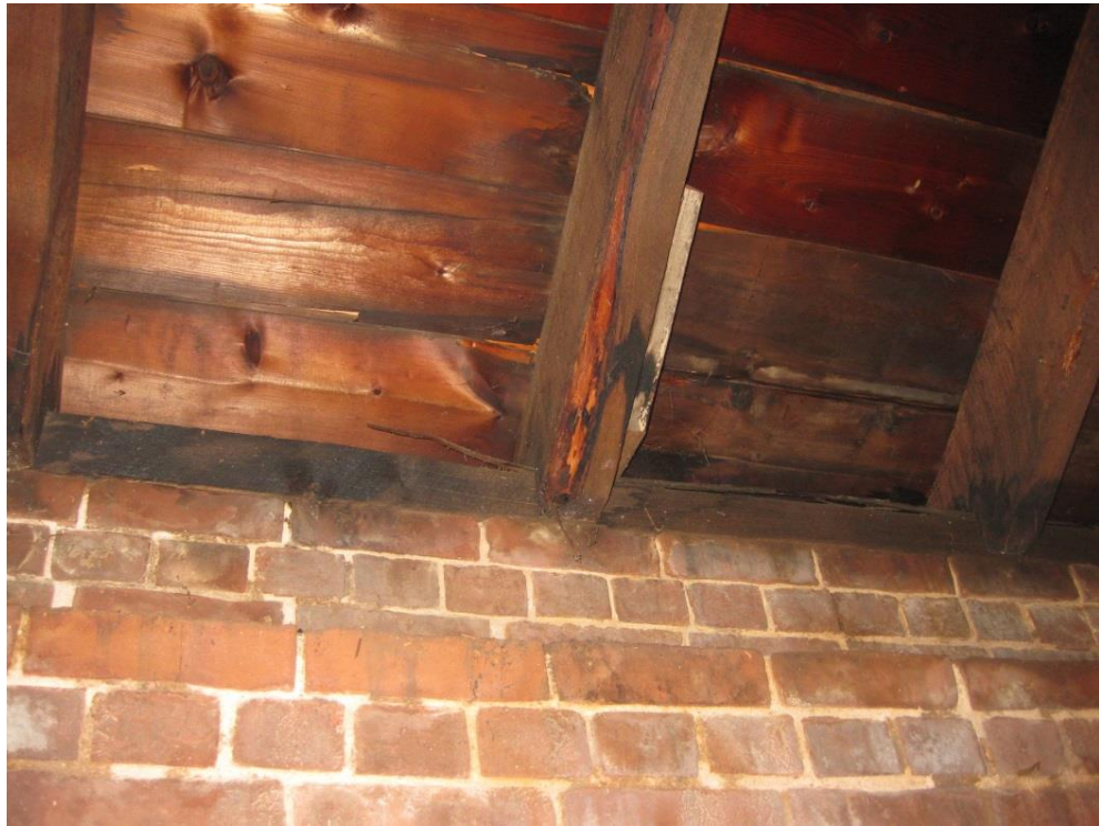
Photo B-11 – Weathered roof planks and cracked rafters
