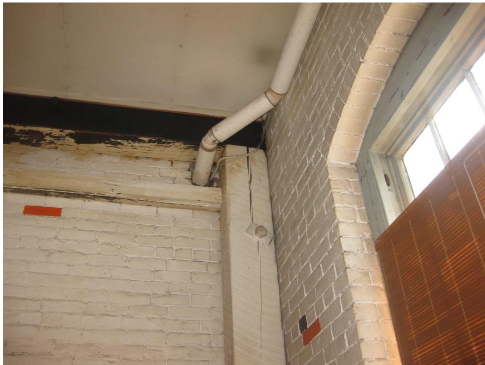
Photo B-14 – Significant vertical crack at wood column
