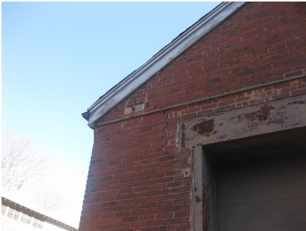
Photo B-8 – Stepped crack at infilled garage door
