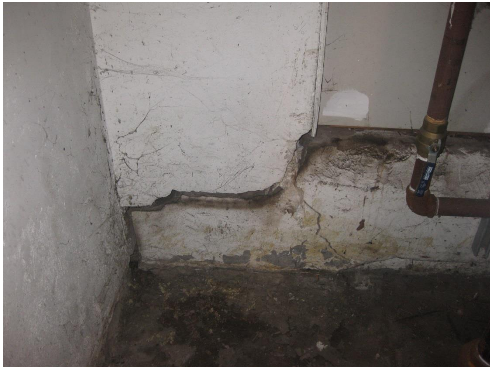
Photo B-2 – Crack at SE corner of Building B at interior face
