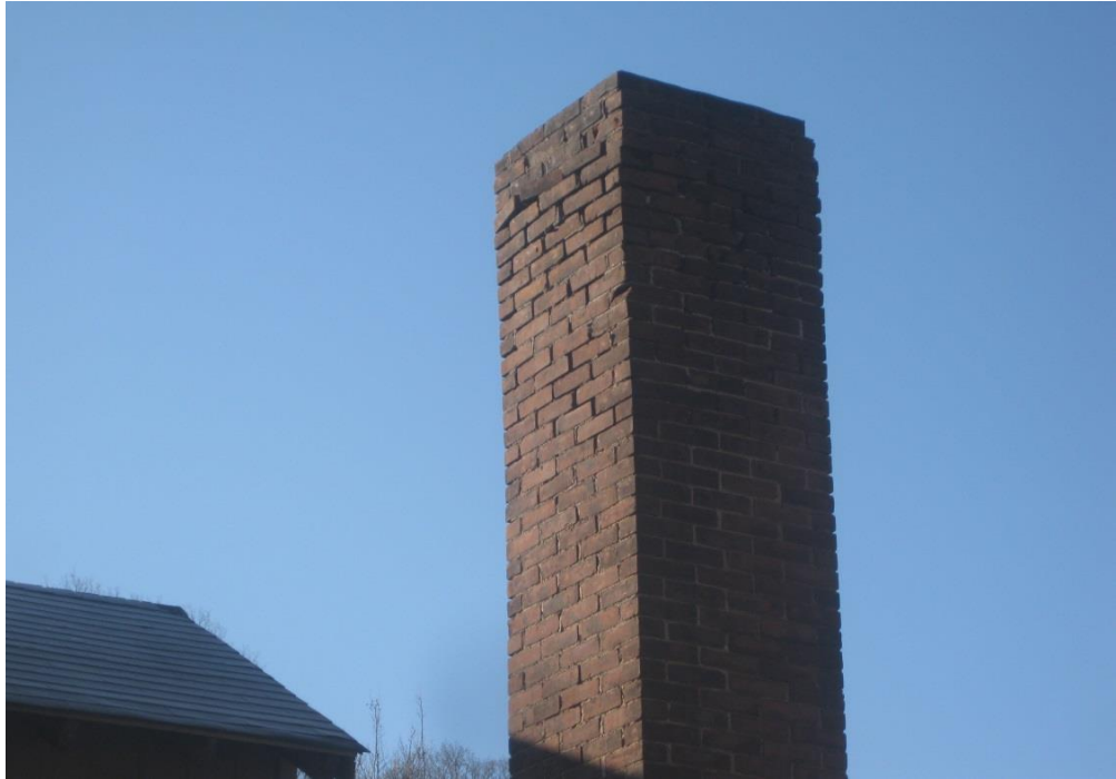
Photo A-5 – Brick degradation at chimney
