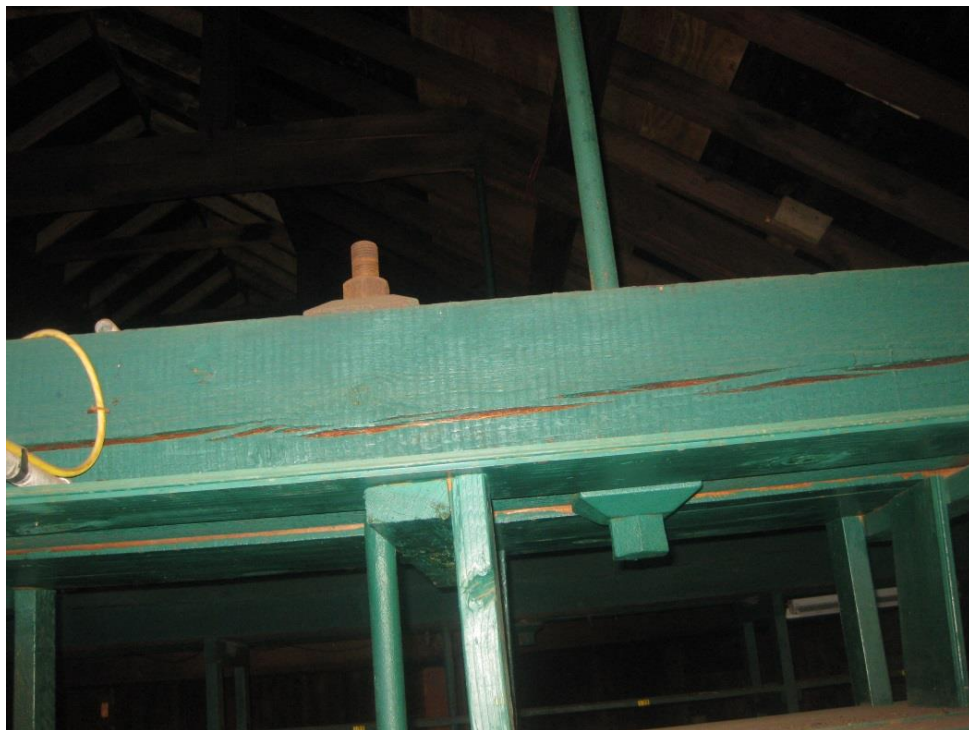
Photo B-16 – Horizontal crack on the wood truss bottom chord (east side)
