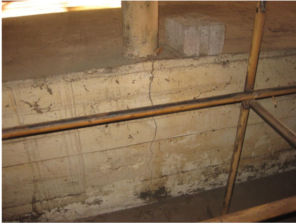
Photo B-13 – Vertical crack at concrete wall directly below column
