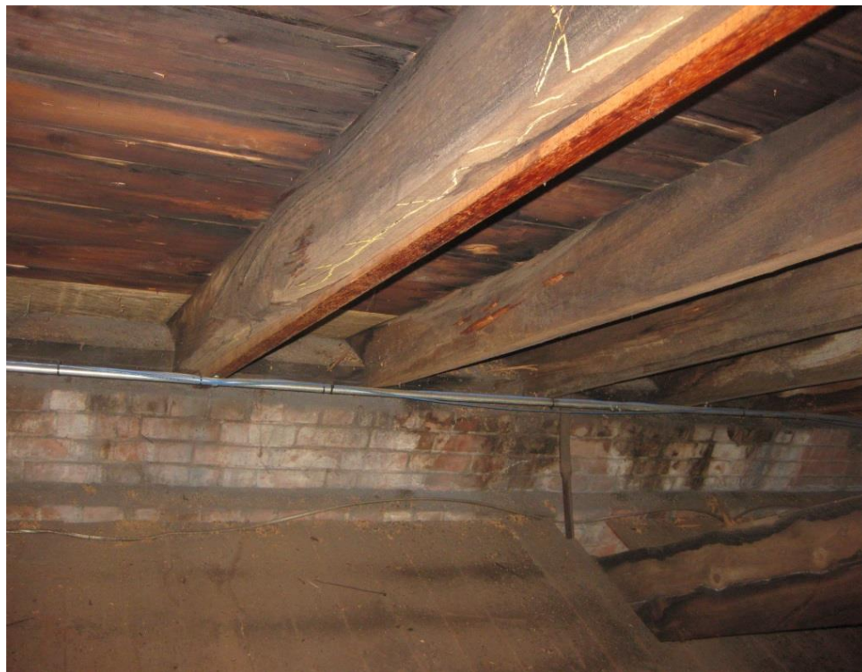
Photo A-18 – Water damage and horizontal cracks at wood rafters
