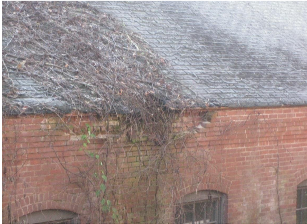
Photo A-7 – Failed roof shingles and exterior brick at north side of Building A
