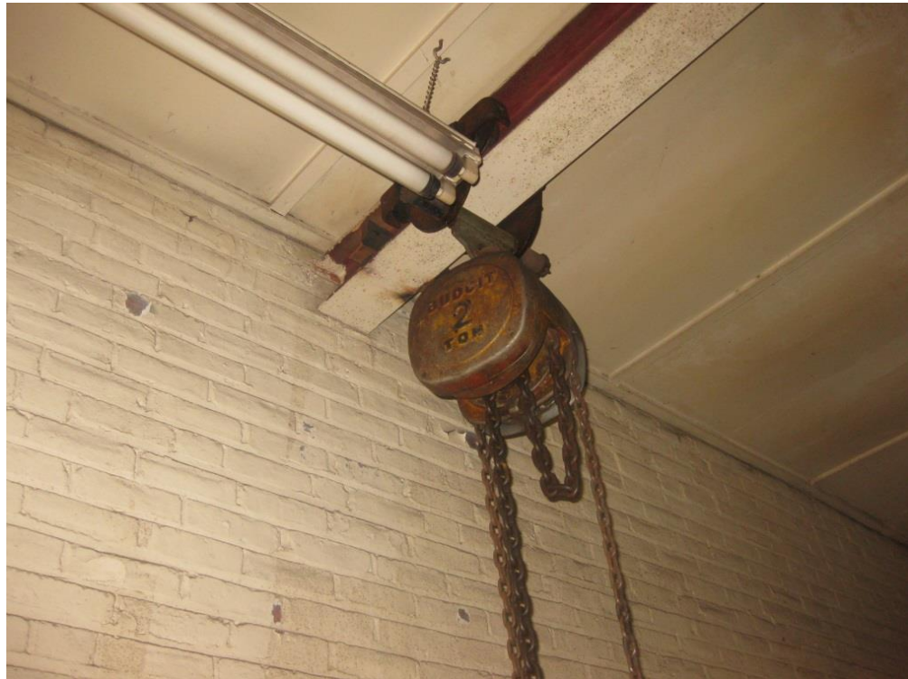
A-21– Two ton chain hoists located in the garage bays
