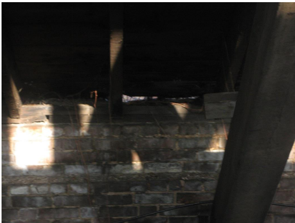
Photo A-20 – Deteriorated wood roof members and planks
