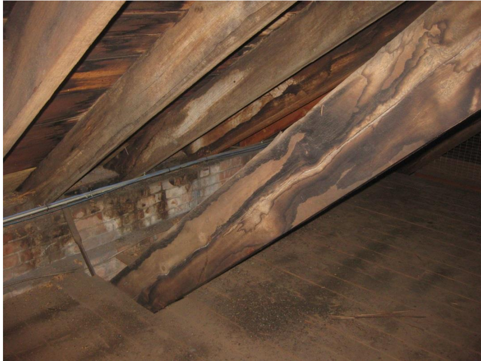
Photo A-17 – Water damage at roof truss and rafters
