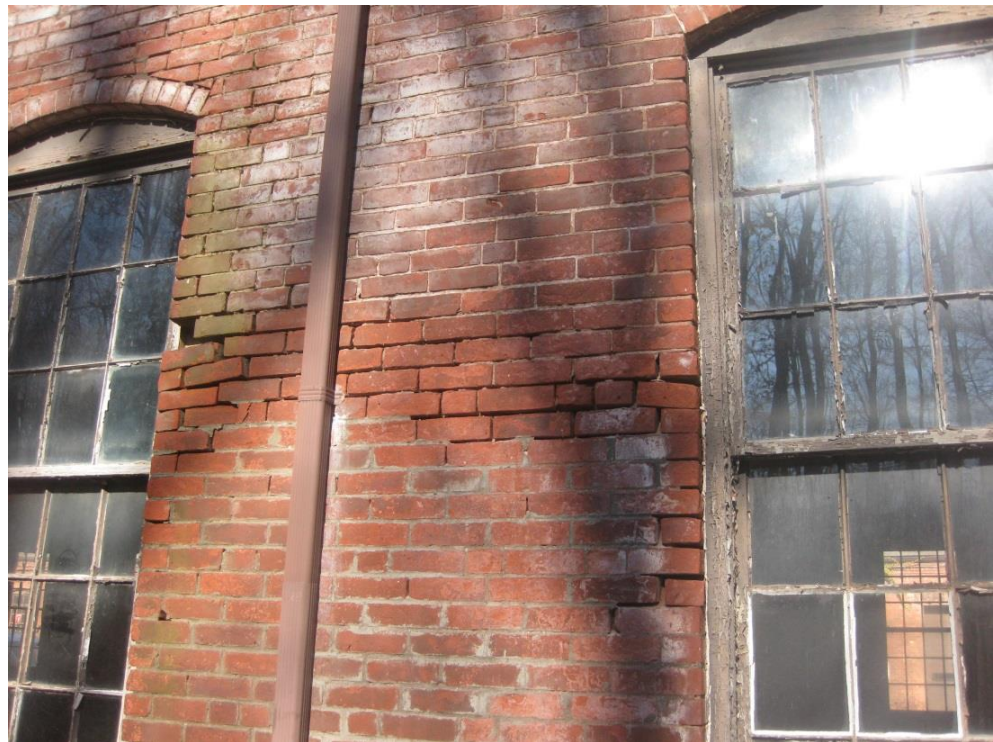
Photo B-4 – Displaced brick and disintegrated mortar at south exterior wall
