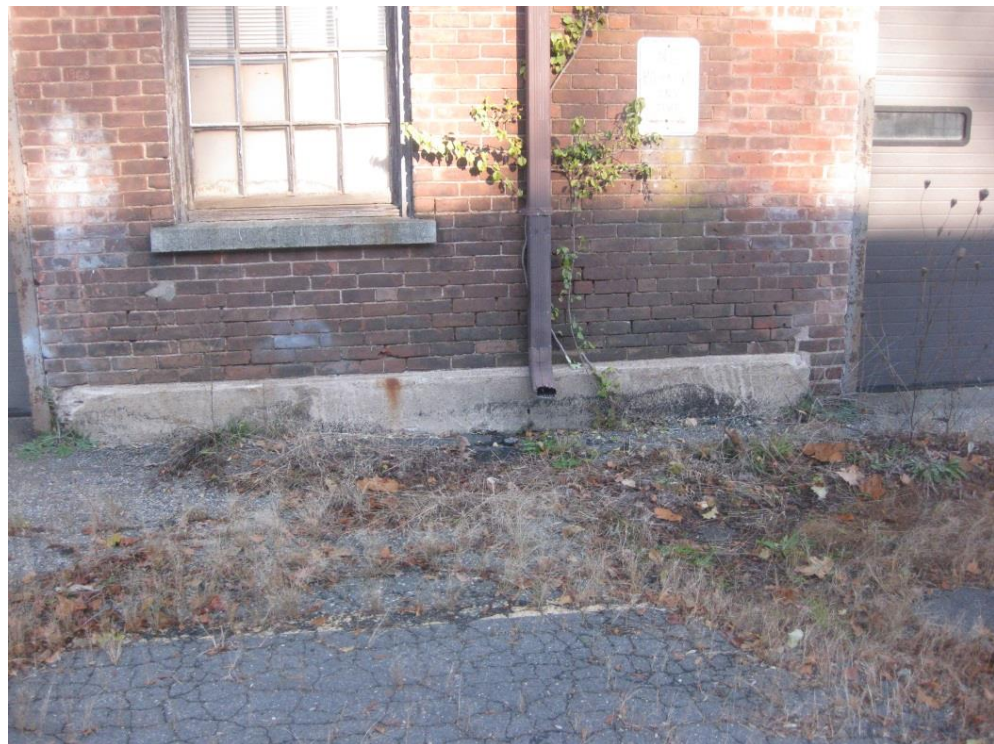
Photo A-10 – Concrete and brick degradation at exterior walls of Building A
