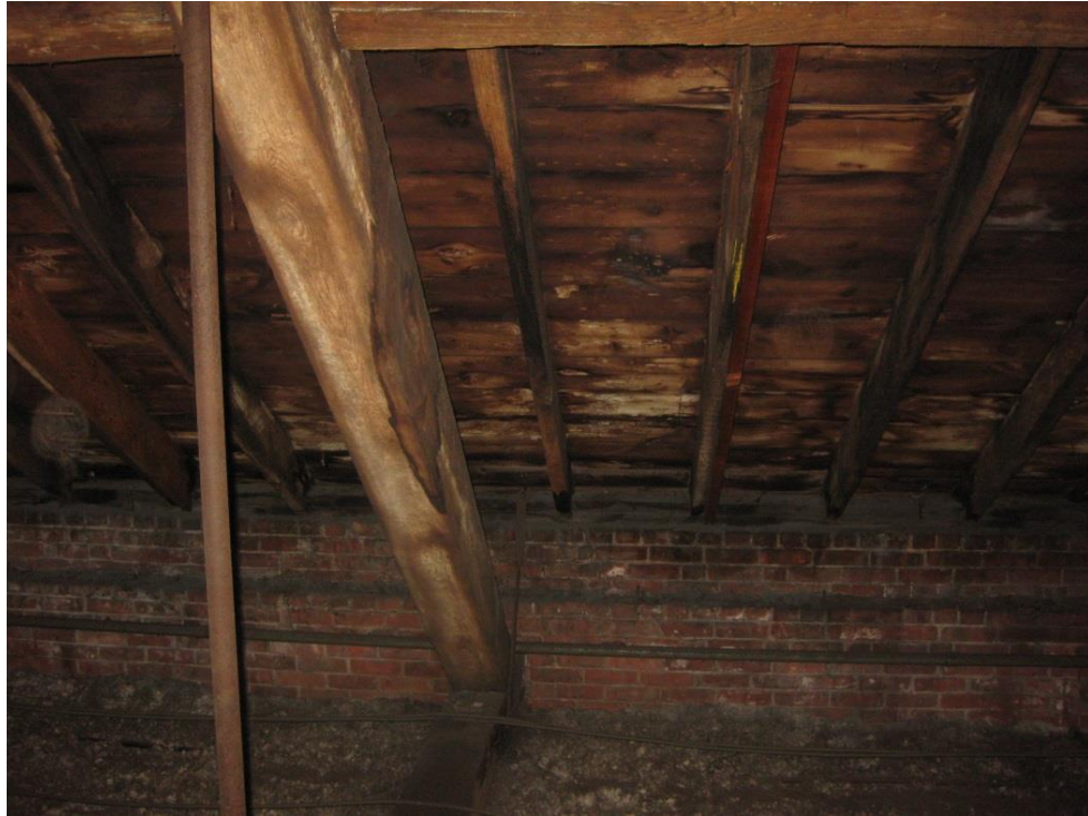
Photo A-19 – Water damage at roof trusses and rafters
