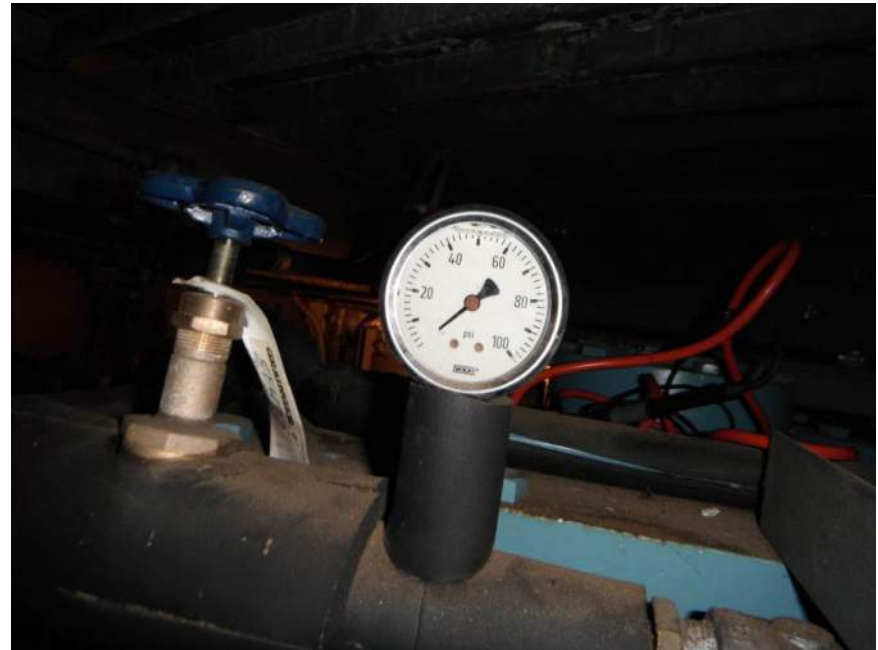
Photo M22: West circulating pump with broken oil pressure gauge
