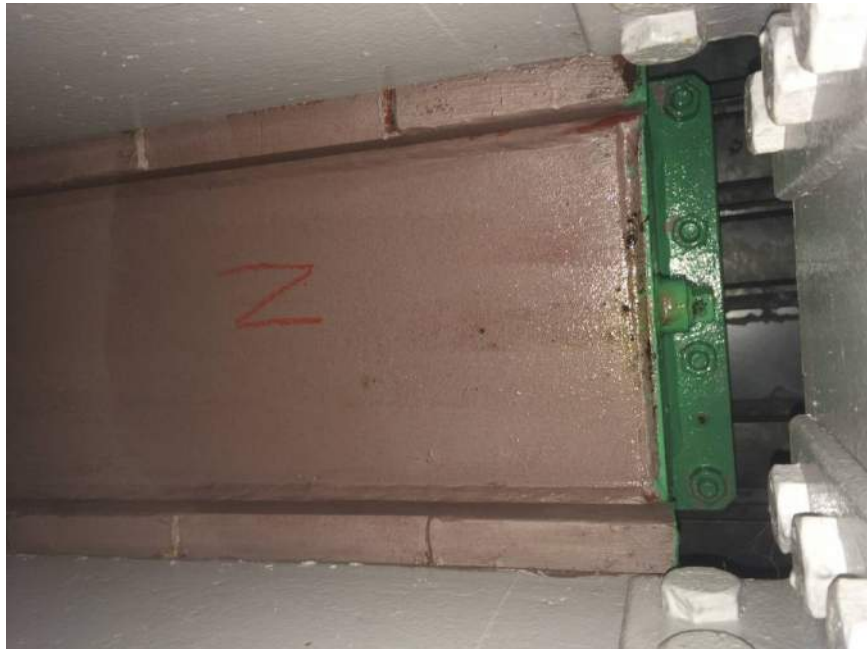
Photo M35: View looking up and south at underside of north center wedge gear reducer. Note presence of primer coat only as noted during prior inspection.
