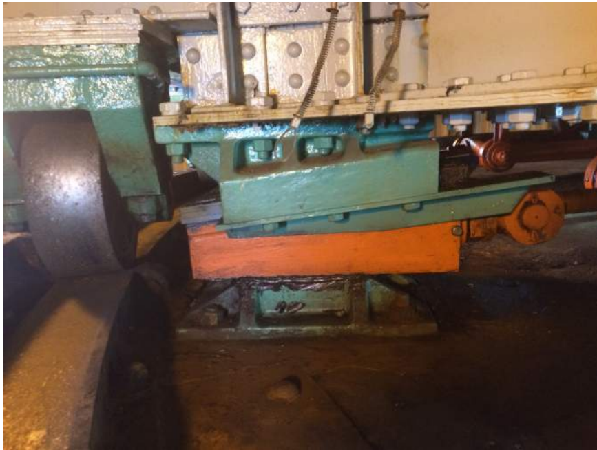
Photo M31: View looking east at SE center wedge assembly.
