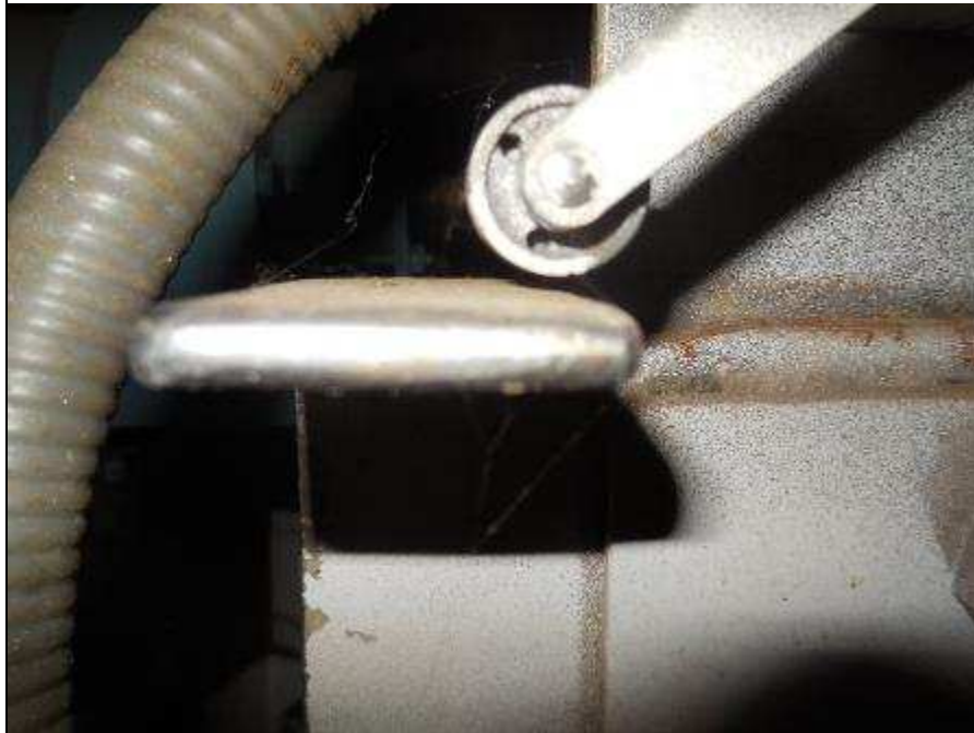
Photo E 5 East Motor Brake Limit Switch
