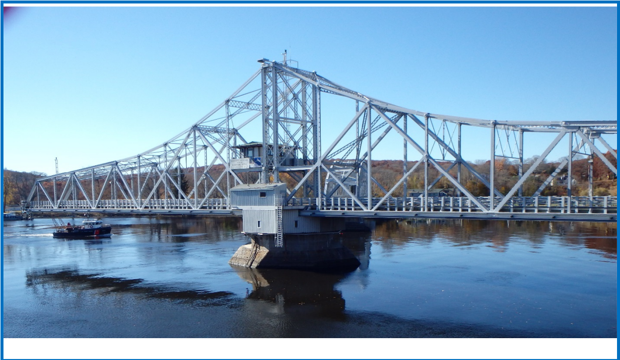
Spans 3 and 4 Swing Span in open position
