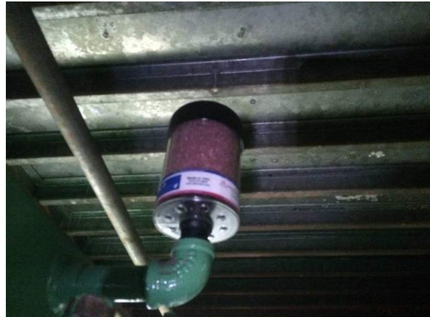
Photo M36: View north center wedge gear reducer desiccant breather. Note all of desiccant has turned pink, indicating the breather should be replaced.
