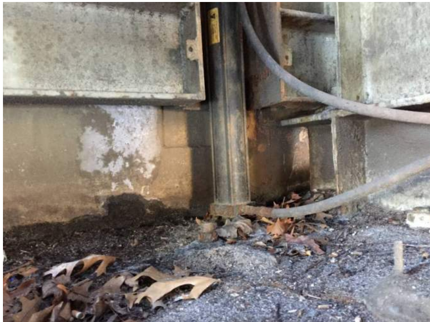
Photo M47: View of NE barrier gate piston with corrosion at base.
