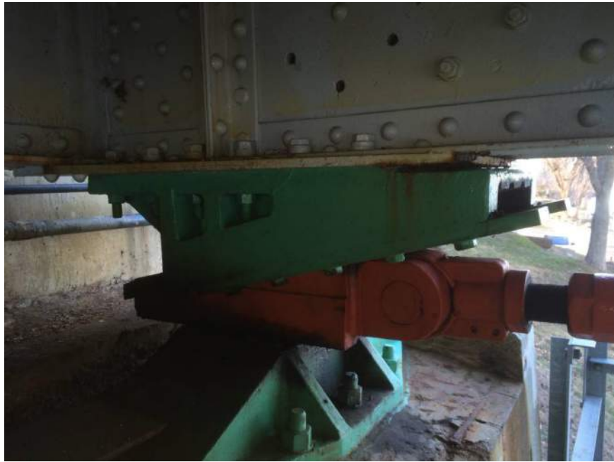
Photo M43: View looking south at SE end wedge assembly. Note corrosion between top shim plate and top shoe.
