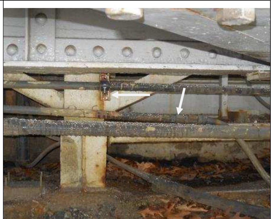
Photo E 10 East Traffic Barrier Gate Hydraulic Feeder Conduit Note that the conduit is not supported.
