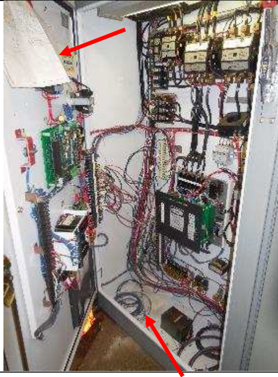
Photo E 7 Drive A Enclosure Interior Note loose wires and paper within enclosure.
