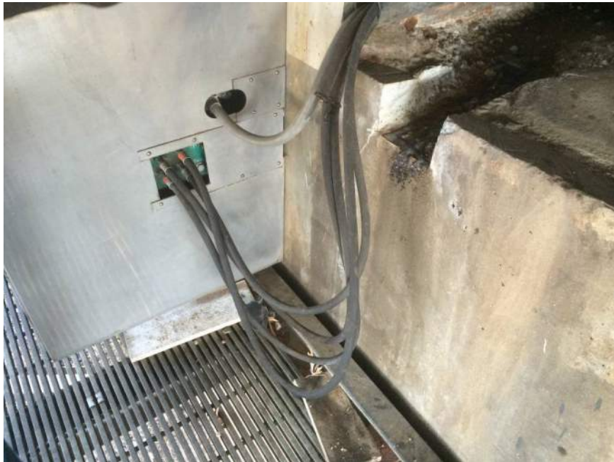
Photo M49: View of W barrier gate hydraulic tubing without heat tracing. Tubing at the west gate can be felt pumping under live load.
