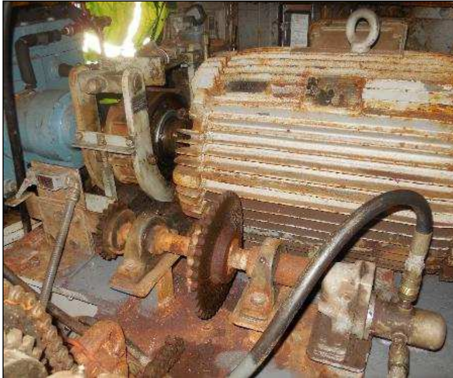
Photo E 1 Typical Span Motor Condition
