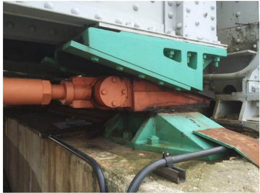
Photo M44: View looking south at NW end wedge assembly.
