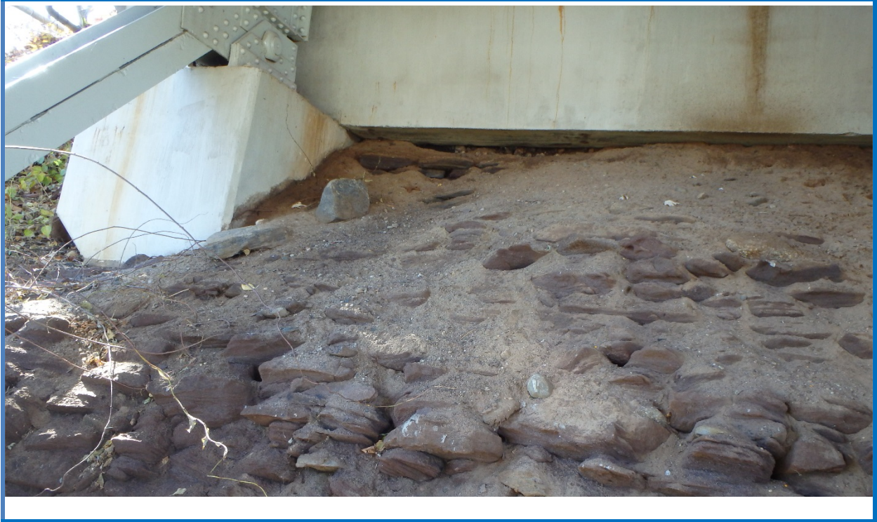
West Abutment. Slope protection in front of spill through abutment and some evidence of erosion.
