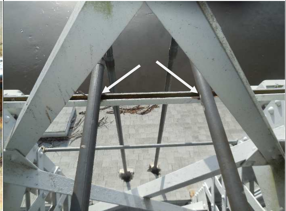
Photo E 26: Control House Platform Conduit To Secondary Resistors
