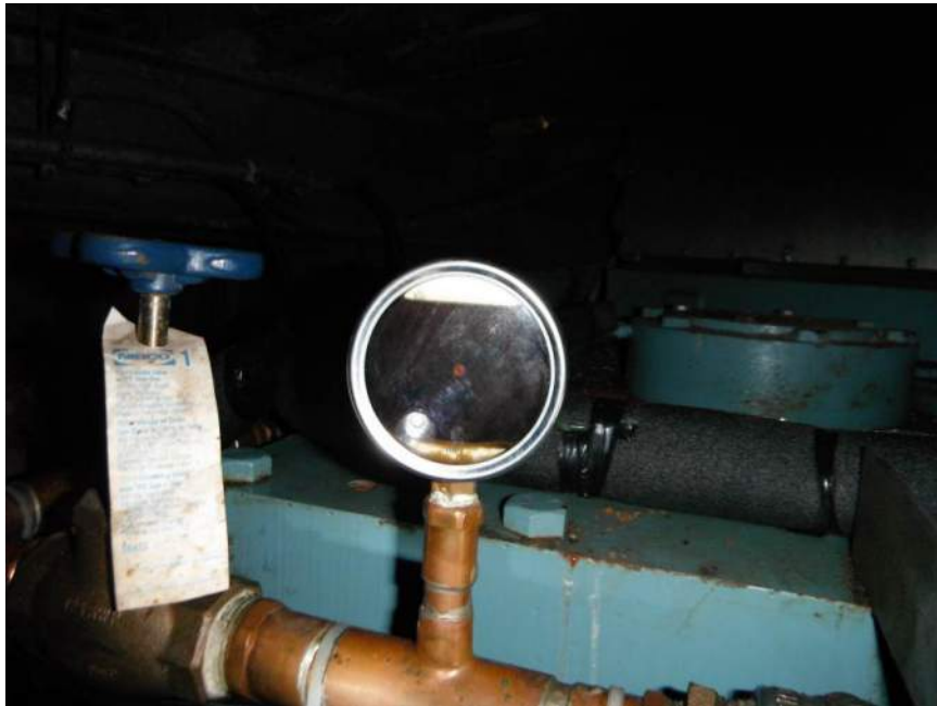
Photo M21: East circulating pump oil gauge with coagulated oil
