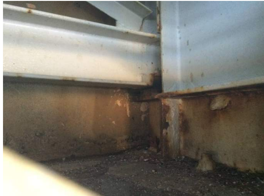
Photo M48: View looking at east barrier gate bottom live load shoe with gap.
