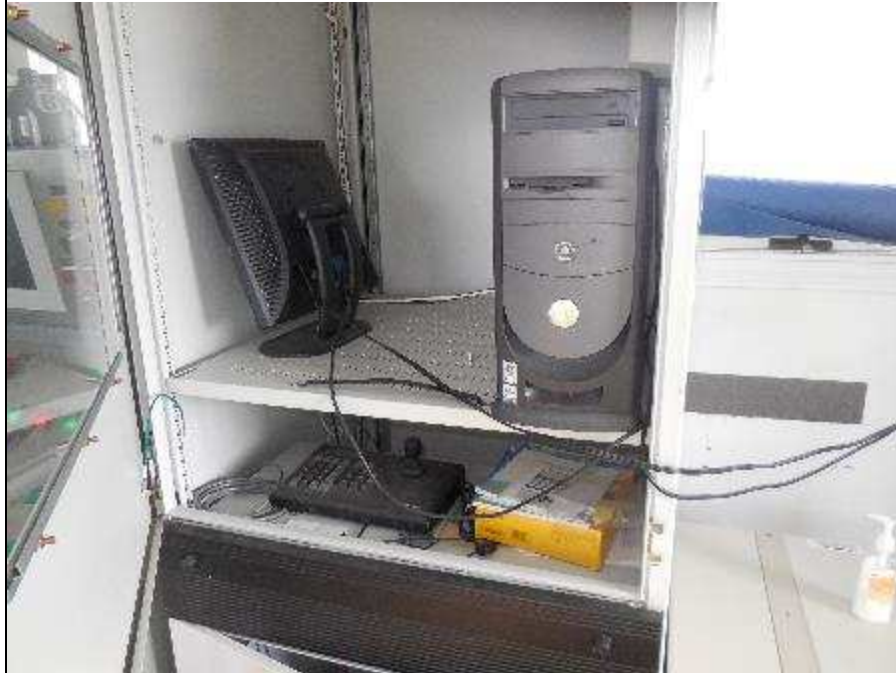
Photo E 11 CCTV Equipment Enclosure Note that cord closes on wires.
