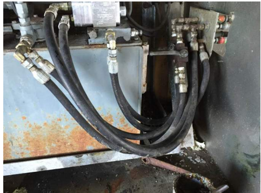
Photo M46: View of W barrier gate hydraulic equipment. Note broken temperature gauge.
