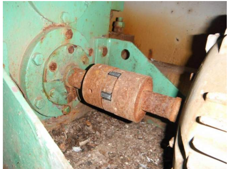
Photo M38: View of north center wedge rotary cam switch jaw coupling. Note lack of paint protection and surface corrosion.
