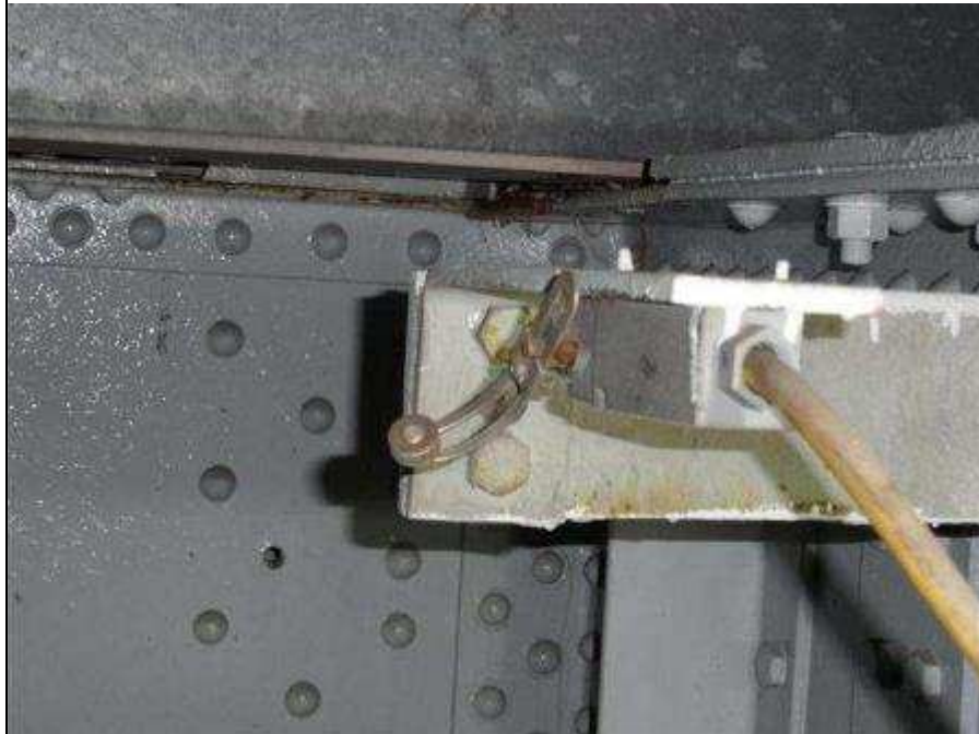
Photo E 3 North Center Wedge Limit Switch Note that the switch arm is bent.
