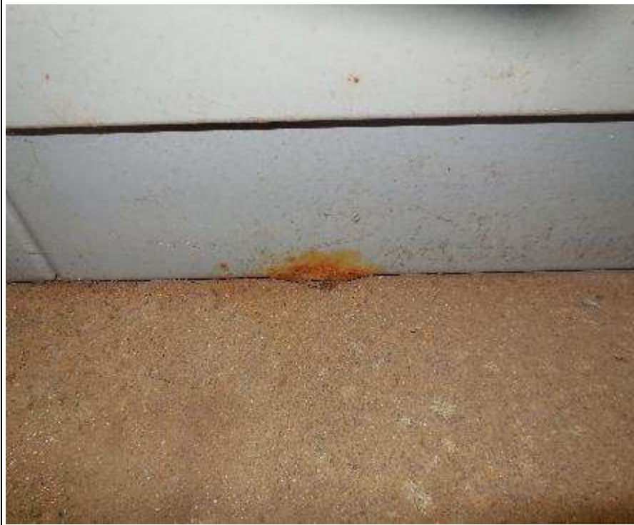
Photo E 19: Bottom of MCC Note corrosion starting to form.
