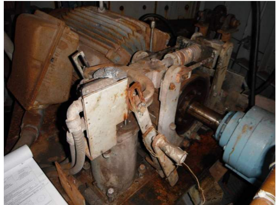
Photo M06: General view of east machinery brake. Note that the manual release lever can no longer be locked in either the engaged or disengaged positions.
