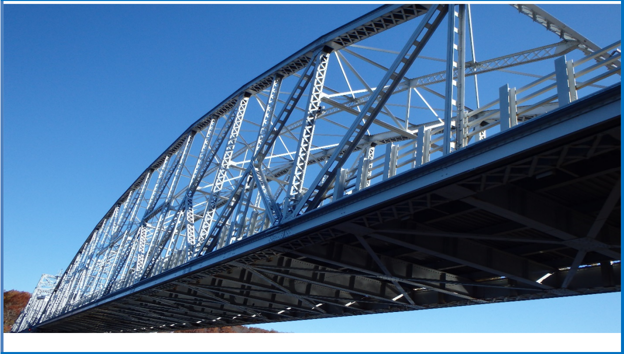
Span 2 Fixed Through Truss North Elevation
