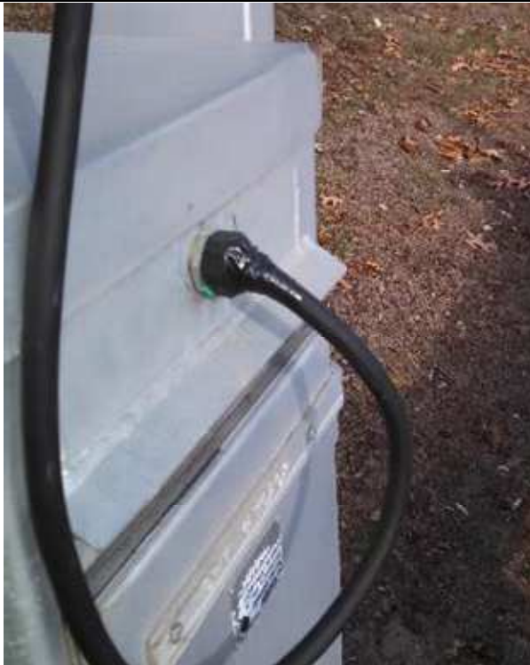
Photo E 9 East Side Oncoming Traffic Gate Note tape over conduit termination.
