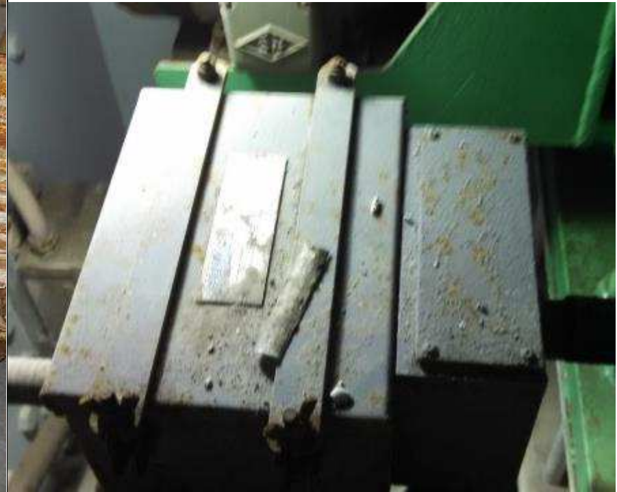
Photo E 2 Typical Rotary Cam Limit Switch Enclosure
