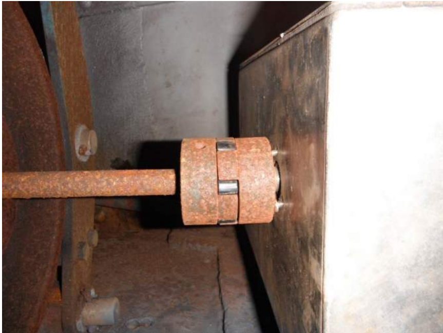
Photo M03: Tachometer / overspeed switch cover screws interfering with coupling
