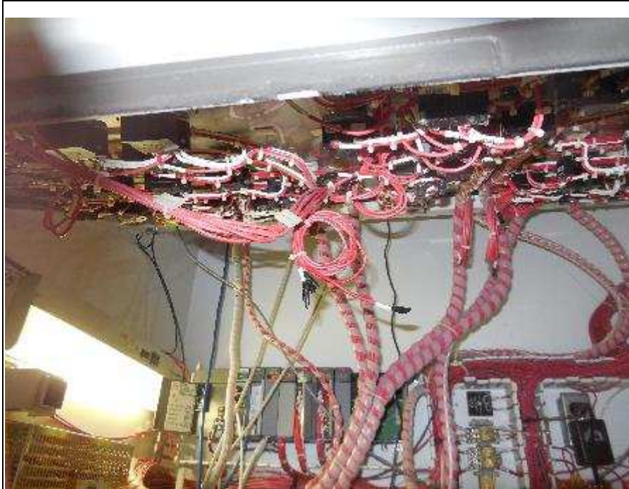
Photo E 15 Below Control Console Note improperly terminated wires
