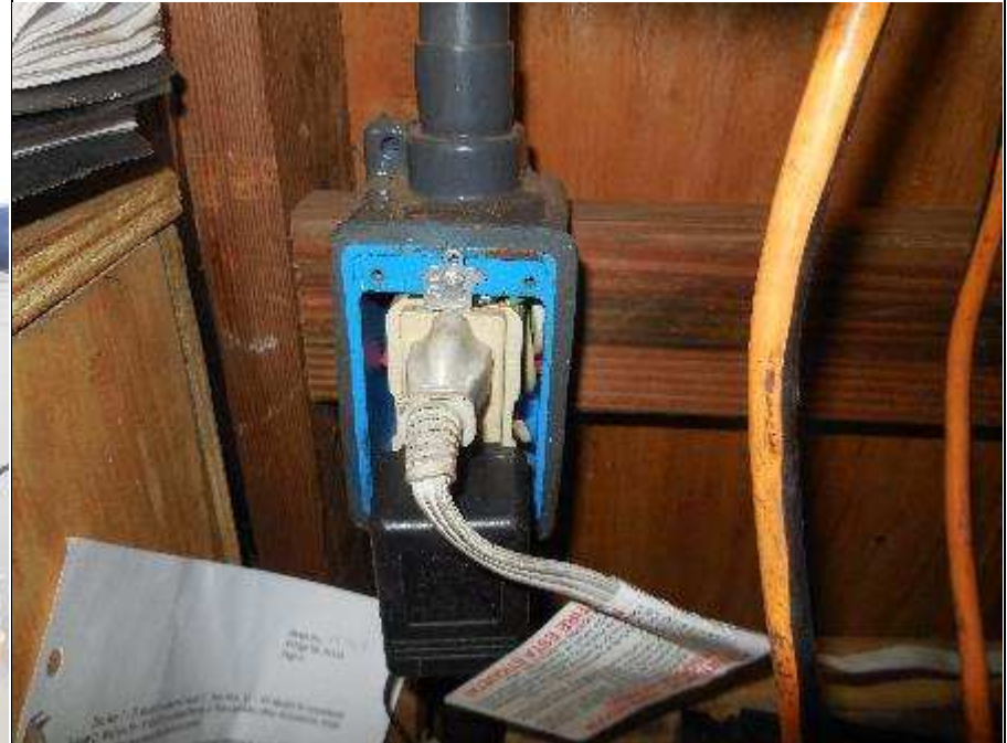
Photo E 12 Receptacle Within Electrical Room Note missing cover plate.
