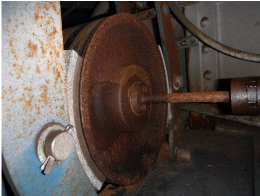
Photo M05: View of west motor rear extension shaft coupled to tachometer/overspeed switch assembly. Note lack of paint protection and light to moderate surface corrosion throughout.
