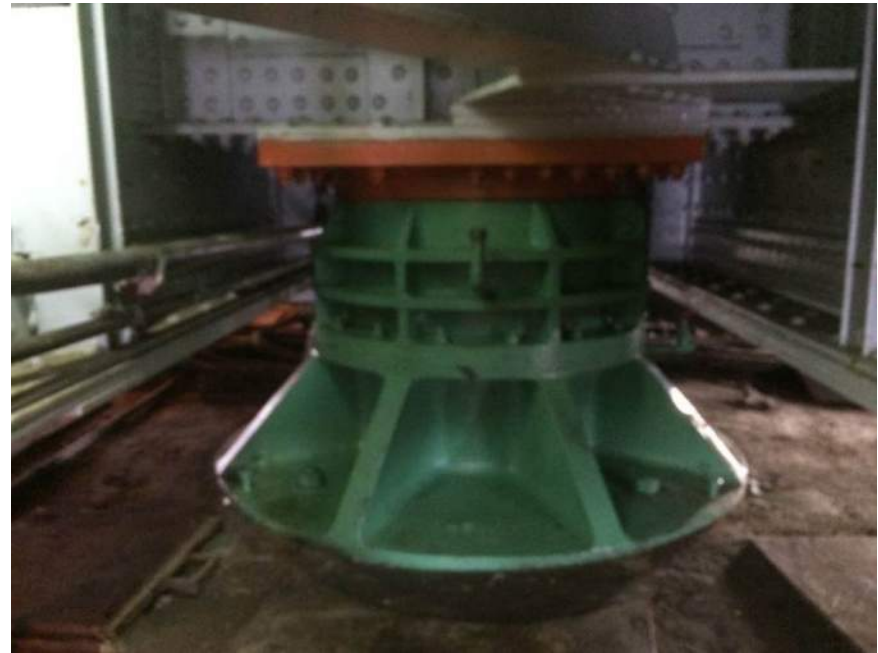
Photo M28: View looking south at center pivot bearing.
