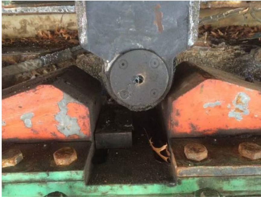
Photo M45: View of east end latch receiver. Note that spring loaded sliding socket blocks are displaced and latch does not fully seat.
