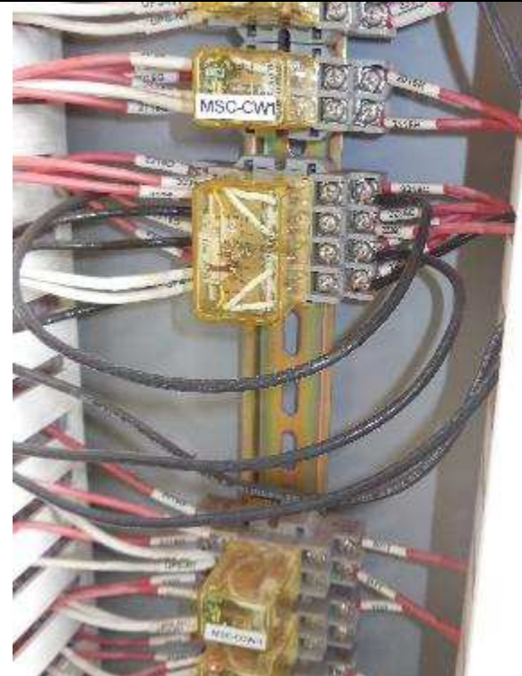
Photo E 16 Inside PLC Cabinet Note bypassed and unlabeled relay
