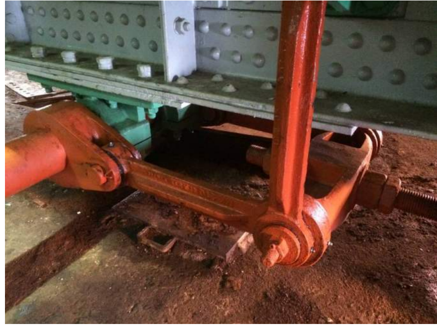
Photo M32: View looking west at NW center wedge lower crank/connecting rod assembly.
