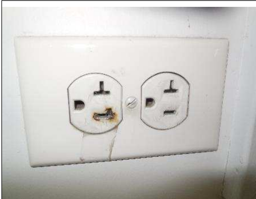
Photo E 13 Receptacle Within Control House Note signs of arcing and overheating.
