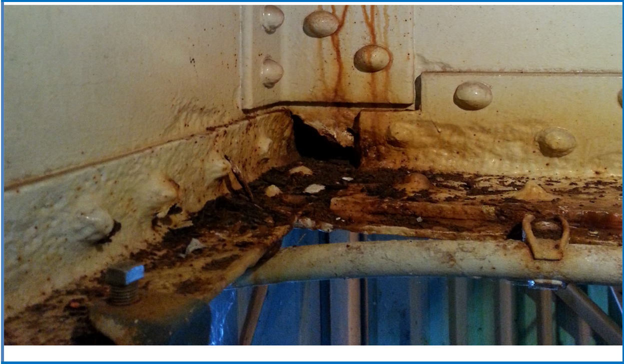
Typical painted over pitting loss in floorbeams and truss members and evidence of additional corrosion.
