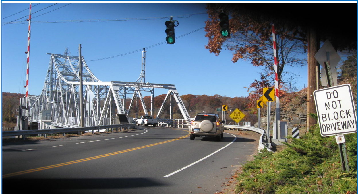
Traffic signals and warning gates in east approach to bridge
