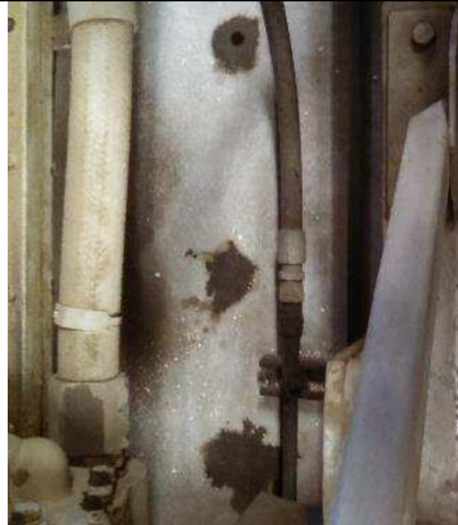
Photo E 22: Generator Note fluid freshly leaked during generator exercising.
