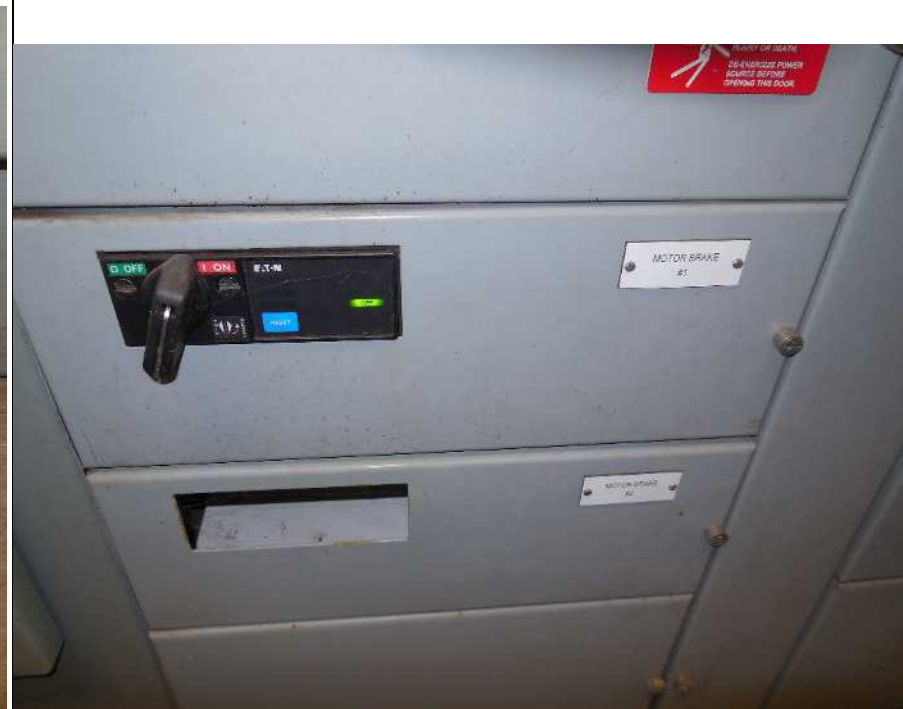
Photo E 20: MCC Note that the motor brake #2 controller is missing.
