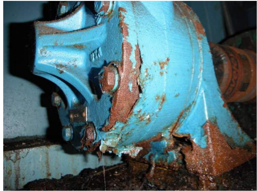
Photo M20: View looking at rear of east speed reducer lubricating oil circulation pump. Note failing paint protection and surface corrosion on both the housing and mounting bolts.
