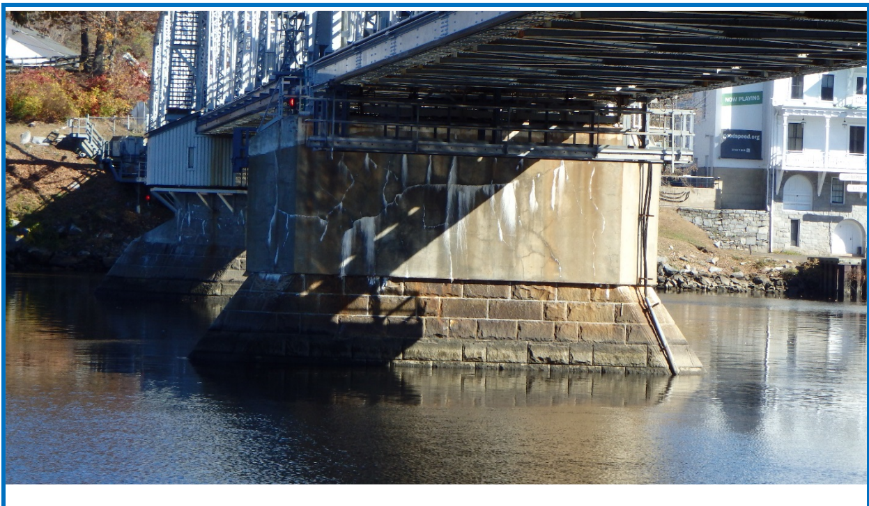
Pier 2 West Elevation. There is extensive map cracking with efflorescence.
