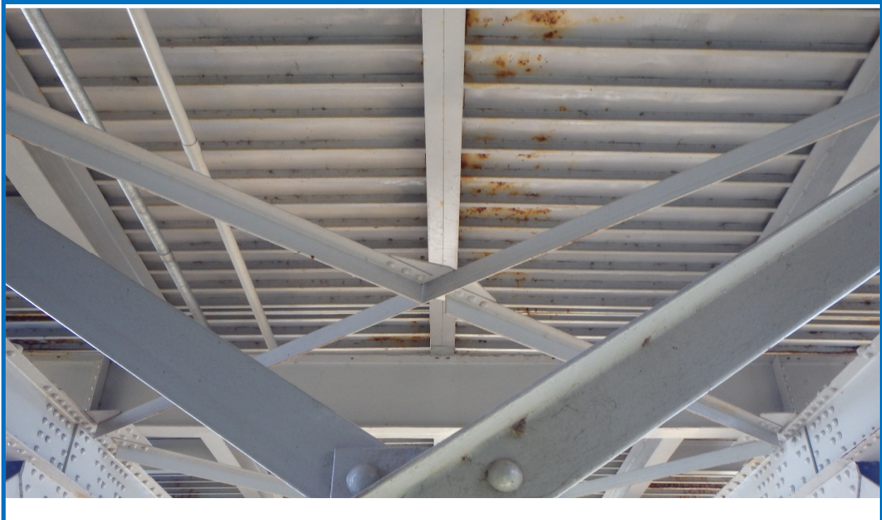
Stay-in-place (SIP) forms cover the deck underside in Spans 1 and 2. Note there are areas of moderate rust on the SIPs.
