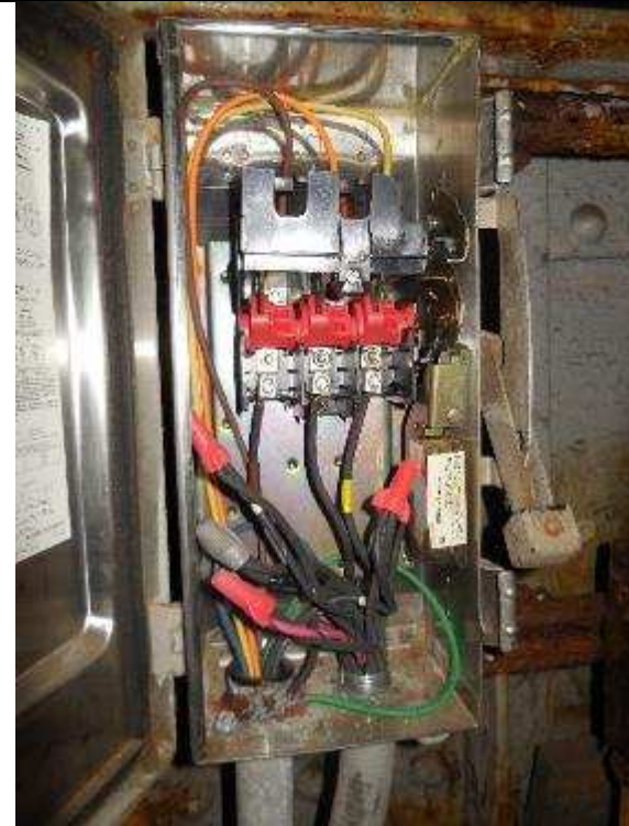
Photo E 8 Center Pier Motor disconnect Switches Note that corrosion on the enclosure, conduit terminals, ground and supports.
