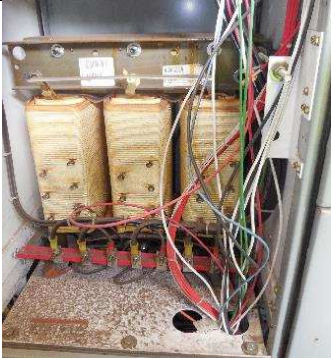
Photo E 21: Lighting Transformer within MCC Note dust accumulation and loose wires.
