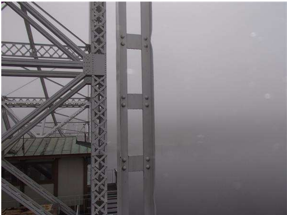
Photo Number: 107 Out-of-plane bending in the vertical member, L9'-U9' of the north truss, span 4 (Construction related).
