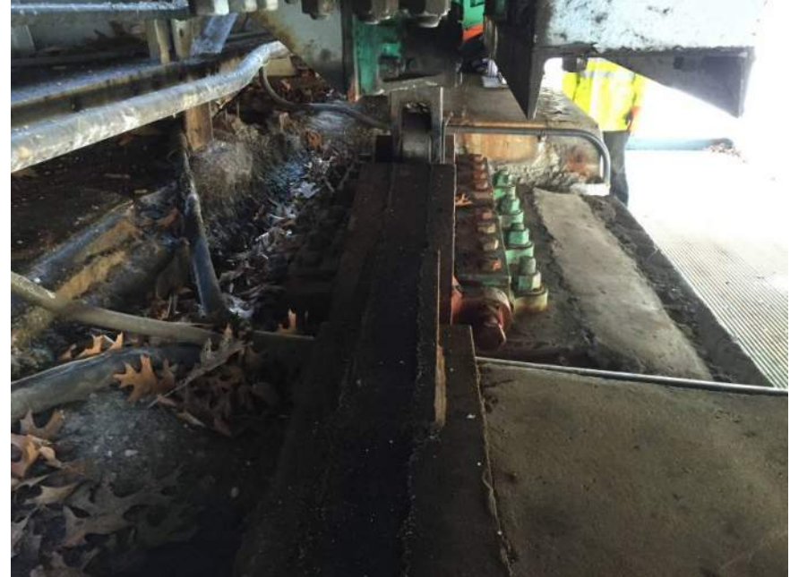
Photo M46: View of east latch not fully seated. Roller on latch follows the steel plates to return back to receiver as the latch does not fully retract to clear the pier prior to the socket blocks.
