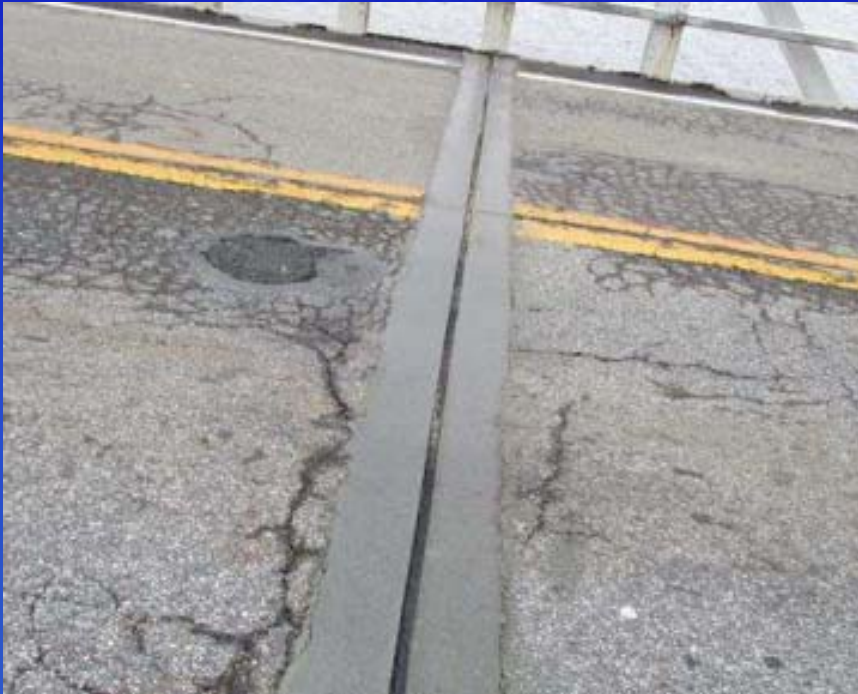
Top of Deck at Span 2 Contraction Joint
