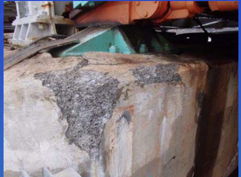
Spall in Pier 2 Cap
