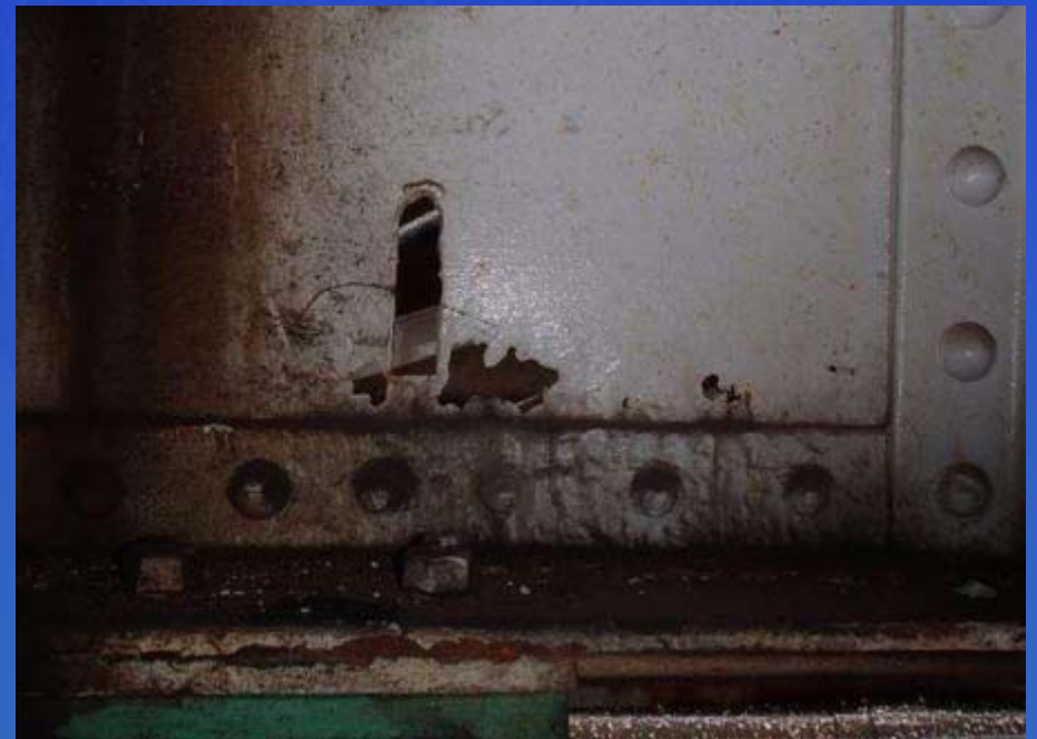
Perforations through Floorbeam Web in Span 4
