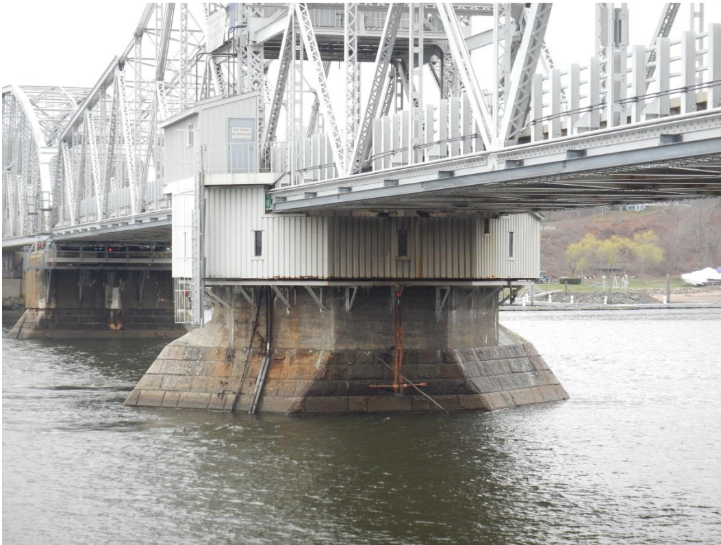
Image 2: An enclosure has been installed on the pivot pier to provide access to and protection for the turning machinery. This marks a visual change to the bridge from its original design, but does not affect the overall historic integrity of the structure.
