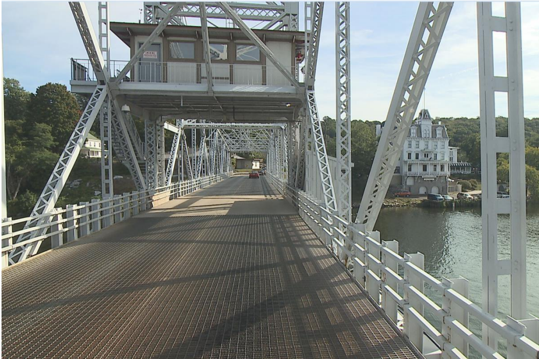
Image 1: Eastbound segment of swing span of portion of the bridge. The driving surface is a steel “singing” grid. The grid is covered beneath the control house to protect the machinery in the swing pier from water intrusion.
