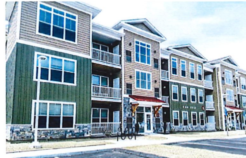
Essex Station Apartment, Essex CT
