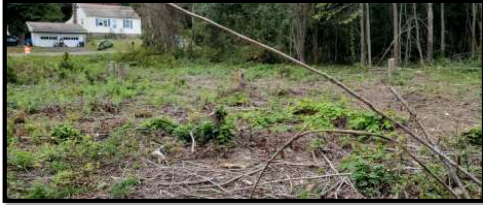
AREA CLEARED FOR STORAGE BINS AND TRAILERS
