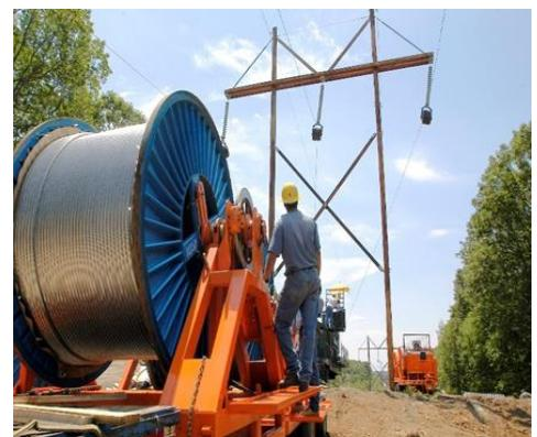
In some locations where helicopters can't fly, we will use bucket trucks set up around the base of each structure and with wire pulling equipment. Pulling sites are set up at various intervals along the right-of-way, typically one to three miles apart. The new wires are pulled through stringing blocks (pulleys) installed at the top of each structure. Once the new wire is strung, the stringing blocks are removed, and the wire is clipped into its final hardware attachment.
