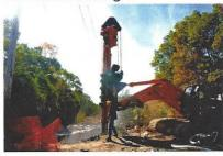
When required, drilling activities usually take place for a few days at each location where structures are being replaced. Depending on soil conditions, the drilling may last longer. The size of the hole will also vary with the size of the new structure and soil conditions. At the end of the work day, any open foundation holes will be safely covered and secured. Once we complete the foundation installation, we will assemble and install the new structures.
