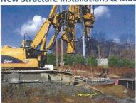
Once the foundations are complete, we'll begin installing the new steel replacement structures. Steel structures often come in sections that are assembled on site. The structure pieces will be delivered to the right of way in advance of this installation process. Cranes and/or bucket trucks are used to lift the structures and set them into position on the foundations.
