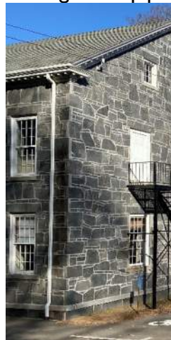
View of roof eave, panel railing, and downspouts.
