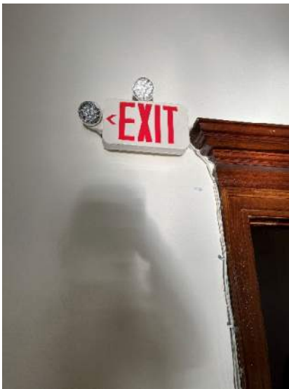
Combination self-contained exit sign
