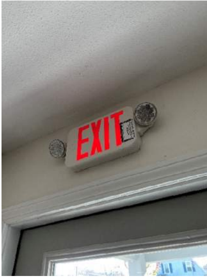
Combination self-contained exit sign
