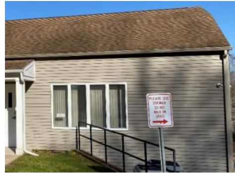
Typical casement windows, south elevation
