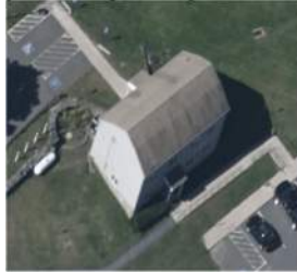
Aerial view of roof
