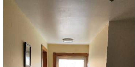
Typical gypsum ceiling at corridor
