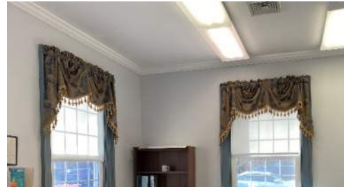
Typical office ceiling
