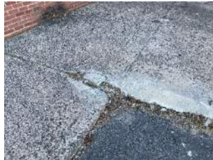
Typical damage at concrete sidewalks
