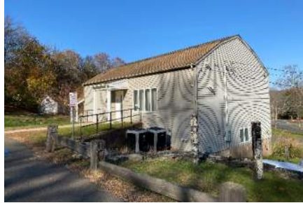
Views of sidewalk to 2 nd floor entry
