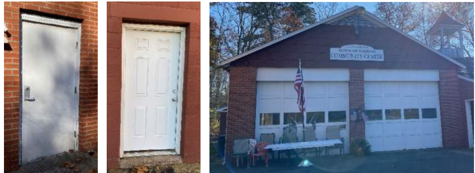
Rear Entry door Side Entry door Garage doors
