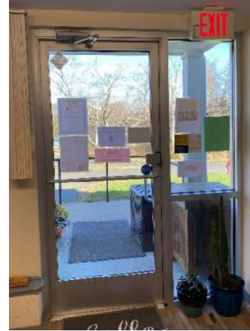
1 st Floor Entry door, interior
