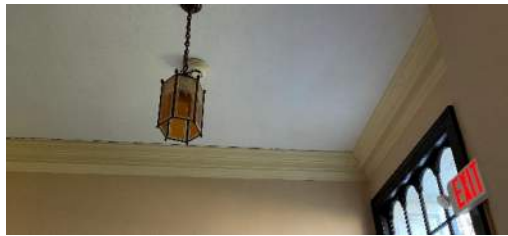
Crown molding in corridors
