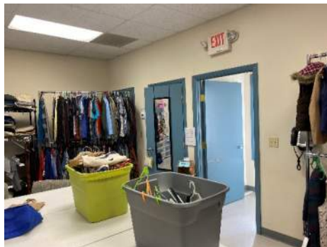
Typical 2 nd Floor wall
