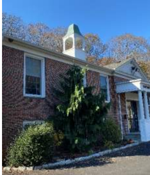
Shrubs at East Elevation
