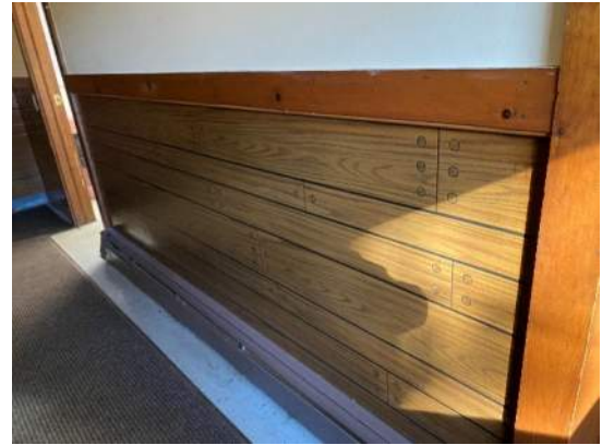
Typical corridor walls
