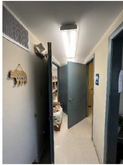
Typical surface linear light fixture
