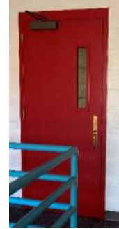
Typical metal door
