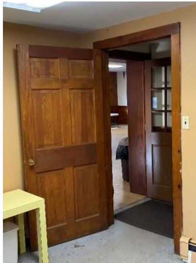
Kitchen interior door
