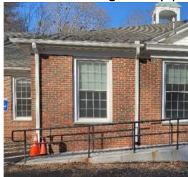
View of roof eaves, gutters, and downspouts.
