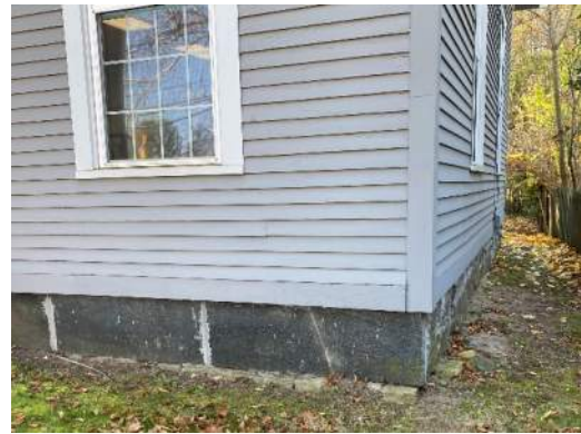
Clapboard siding
