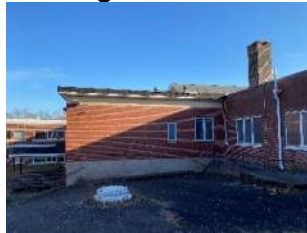
Typical asphalt paving at rear of school
