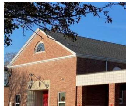
Asphalt roof at old entry
