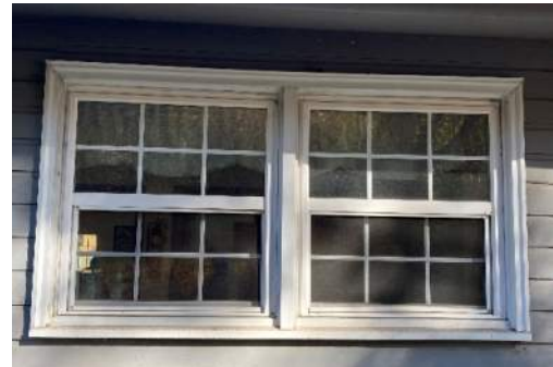
Double hung windows at Kitchen
