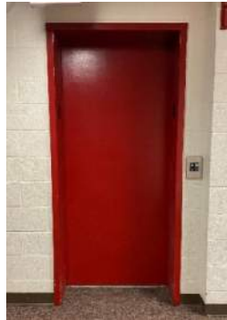
Elevator door at 2 nd Floor
