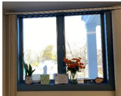
Typical casement window, interior
