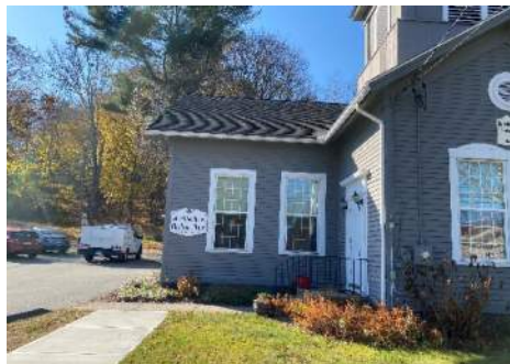
Shrubs at North Elevation
