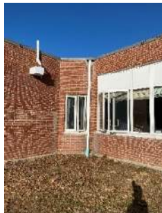
Staining at rain leaders and window sills
