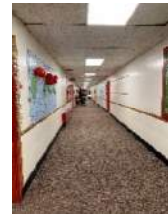
Gypsum board walls in west wing
