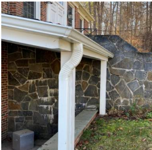
Retaining wall at North Elevation
