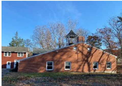
Exterior – West elevation
