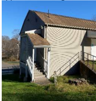
2 nd Floor egress stair
