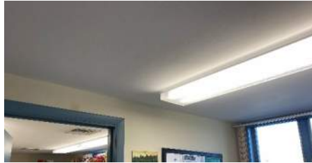
1 st Floor gypsum board ceiling
