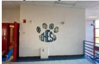
Typical CMU wall
