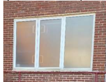
Typical toilet room windows
