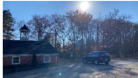
View of parking lot from Candlewood Hill Road
