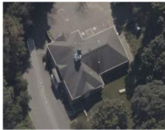
Aerial view of roof
