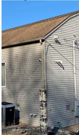
View of roof eave, gutters, and downspouts.
