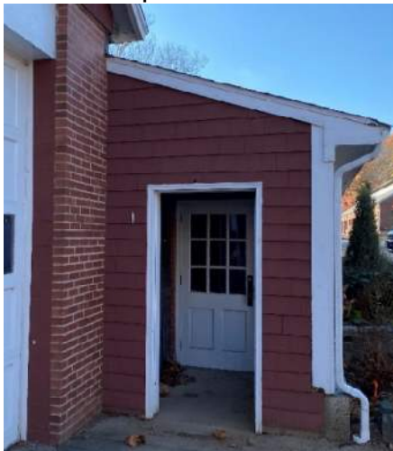
Front Entry vestibule
