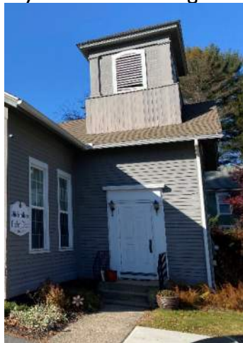
Original exterior doors
