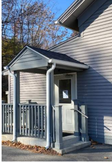
Main Entry door, exterior
