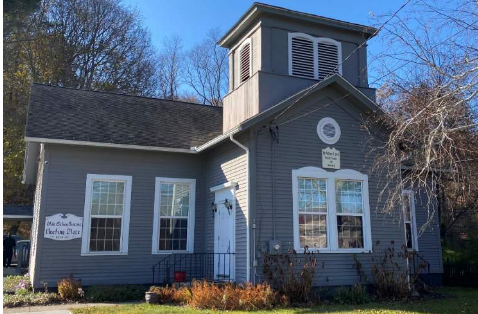
Double hung windows at front and sides
