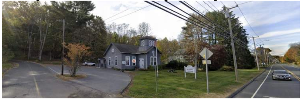
Street view looking north
