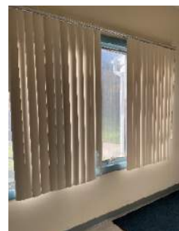
Typical casement window, interior
