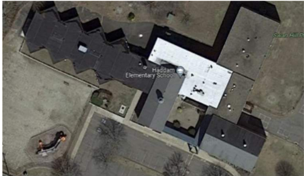
Aerial of roofs
