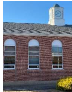
Staining at rain leaders and window sills
