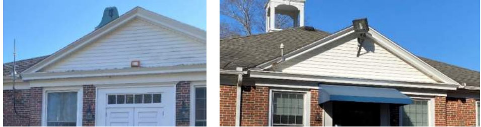
Vinyl sided gabled ends
