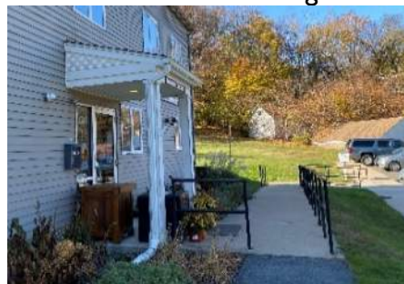
ADA ramp at building entry
