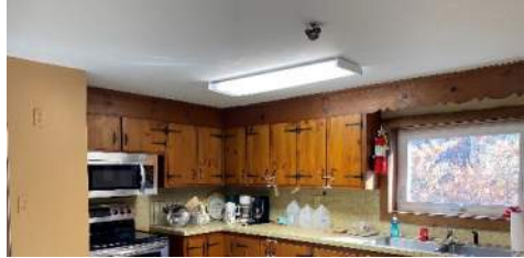
Gypsum board kitchen ceiling
