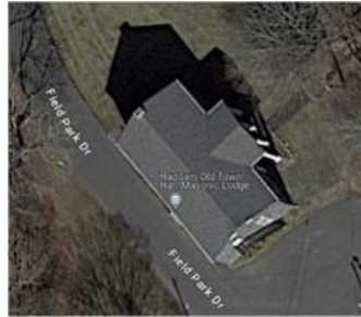
Aerial view of roof
