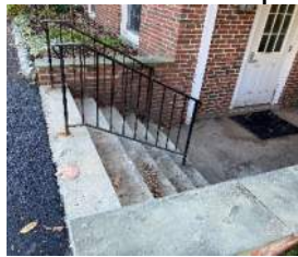
Steps at north lower level entry
