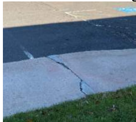
Cracks in various concrete sidewalks
