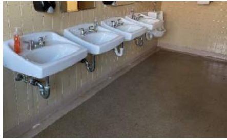
West wing epoxy flooring in Toilet Rooms
