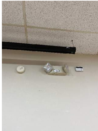
Typical self-contained emergency light
