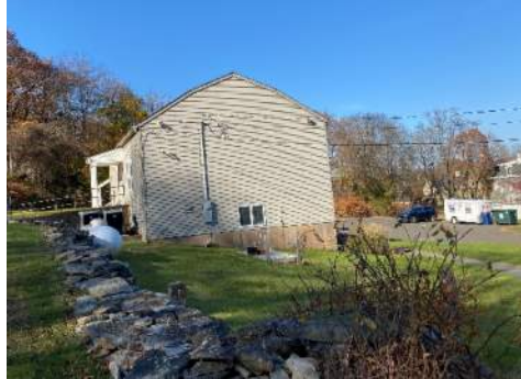
Stone retaining wall
