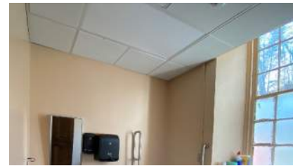
ACT ceiling in toilet room
