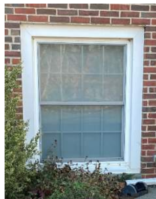
Typical 8/8 double hung at basement level
