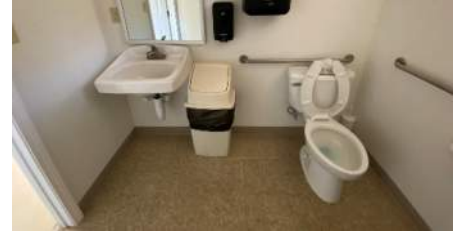
Typical VCT flooring in toilet rooms
