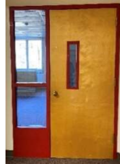
Typical classroom and library door
