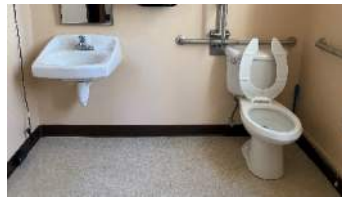
ViCT flooring in toilet room
