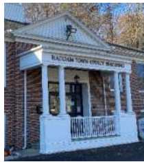
Front entry porch
