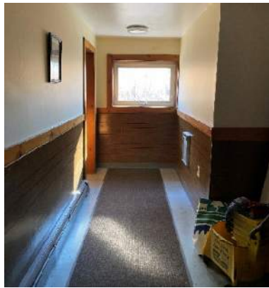
Typical corridor walls
