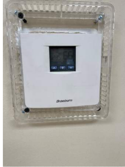
Typical stand alone thermostat
