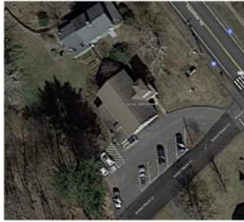
Aerial view of roof
