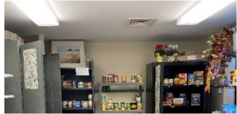
1 st Floor gypsum board ceiling
