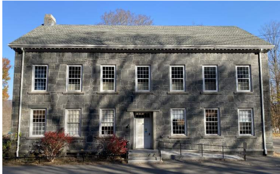
Exterior – West elevation
