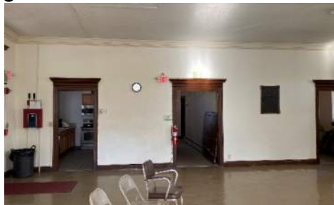
Typical Meeting Room wall
