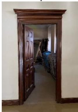
8 Panel historic door and trim
