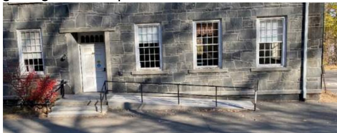
Front entry ramp
