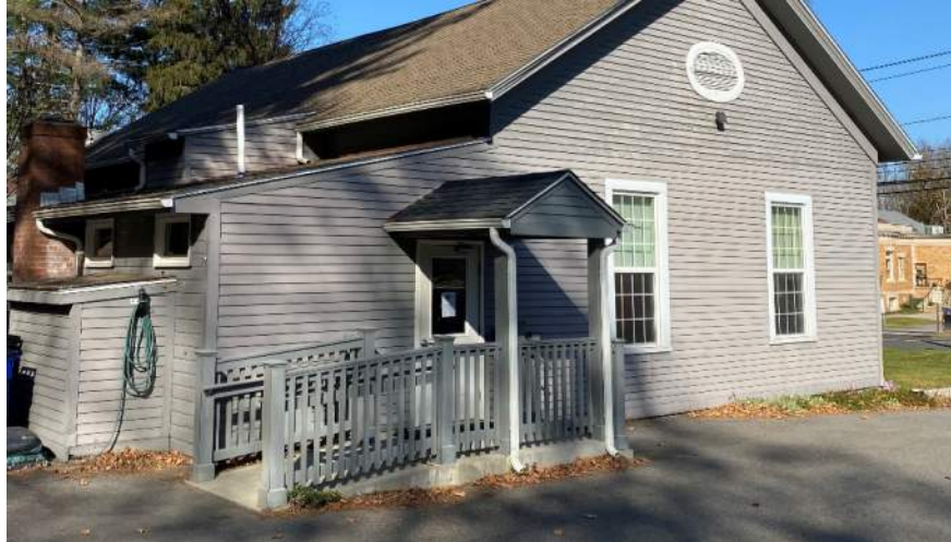
Accessible ramp entrance
