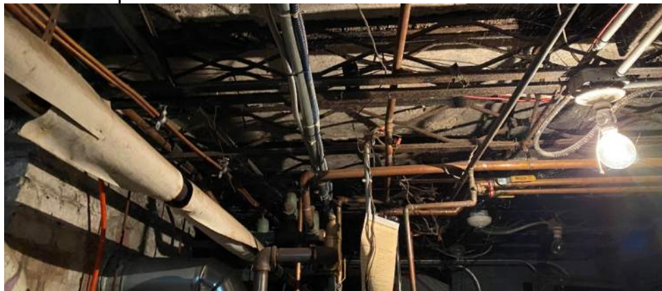
Basement ceiling structure
