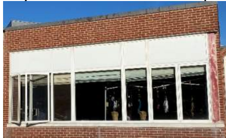
Typical classroom windows
