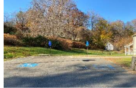
ADA spaces – upper lot
