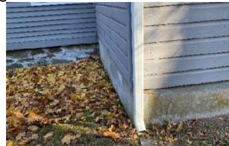
Newer concrete foundation
