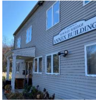
Typical casement windows, north elevation
