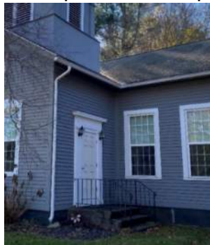
View of roof eave and gutters
