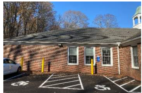
ADA accessible parking
