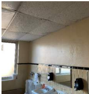
West wing toilet room
