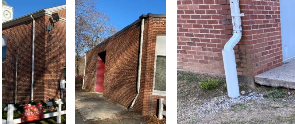
View of roof eave, downspouts, and underground connections
