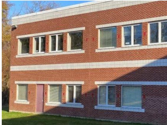
Typical windows, east wing
