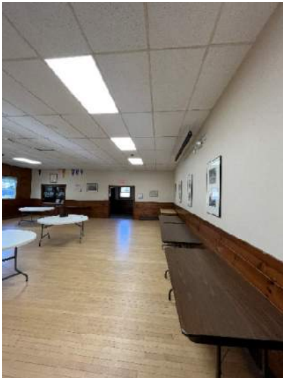
Typical 2'x4' recessed light fixtures
