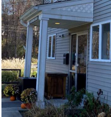
1 st Floor Entry door, exterior
