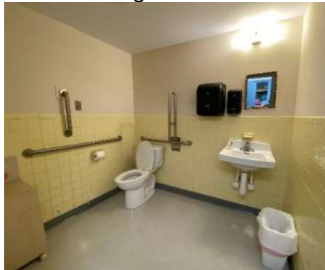
1 st Floor toilet room
