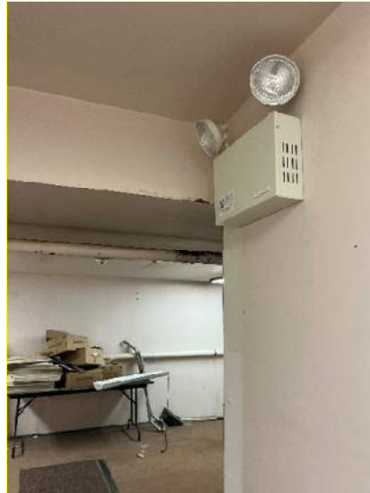
Typical self-contained emergency light
