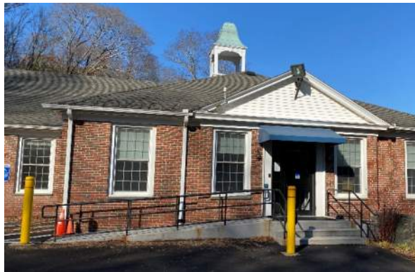
South accessible entrance, exterior
