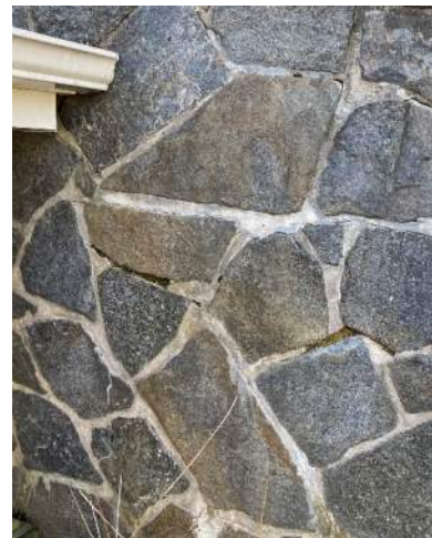
Missing mortar
