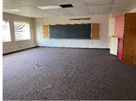
Typical classroom, east wing
