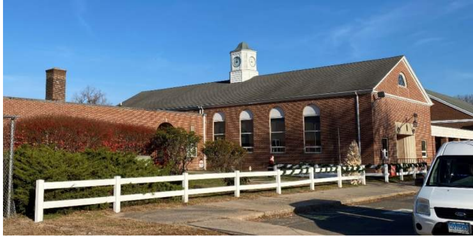
Typical fencing and landscaping at west wing
