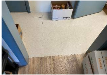
1 st Floor VCT in corridor
