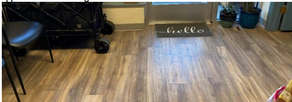
Typical 1 st floor LVT flooring
