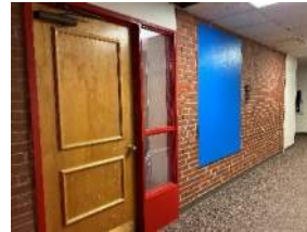
Brick wall in east wing
