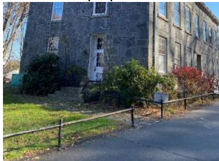
Shrubs at North Elevation
