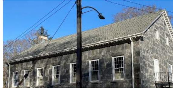
Asphalt shingle roof
