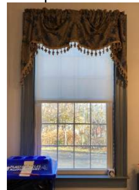
Typical 12/12 double hung 1 st Floor
