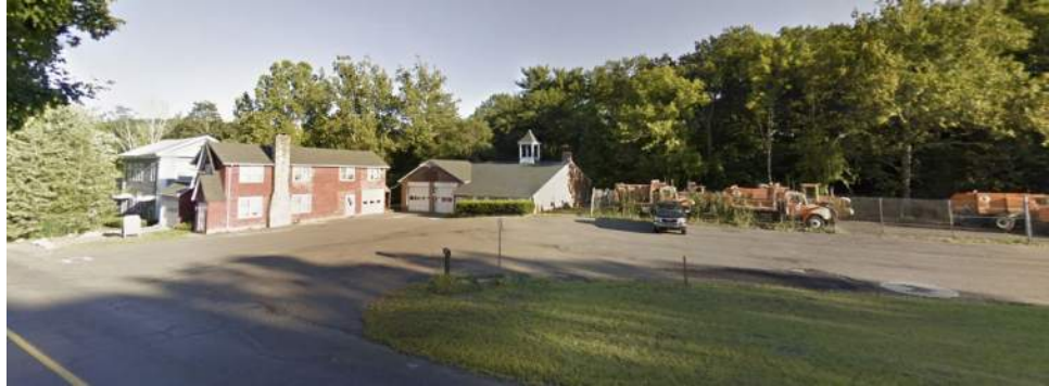
View looking east
