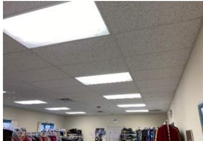
2 nd Floor ACT ceiling
