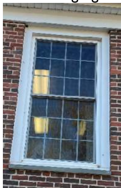
Typical 12/12 double hung Window, exterior
