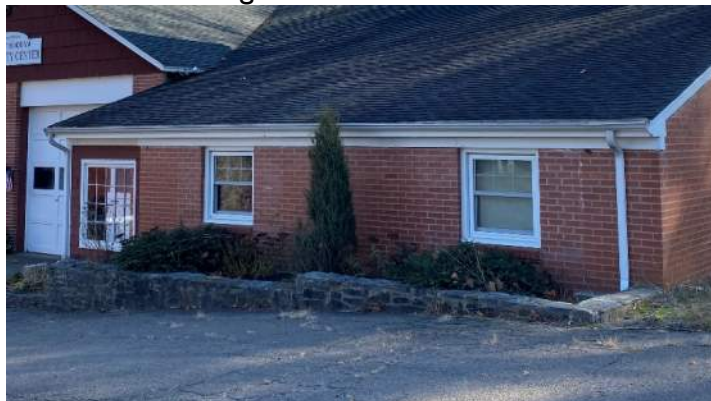
Shrubs at North Elevation
