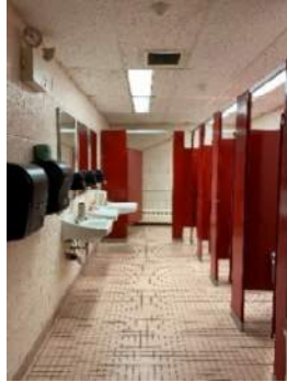
East wing toilet room
