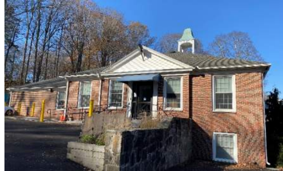
Retaining wall at South Elevation
