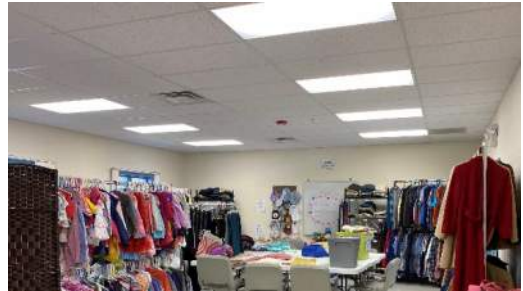
2 nd Floor ACT ceiling
