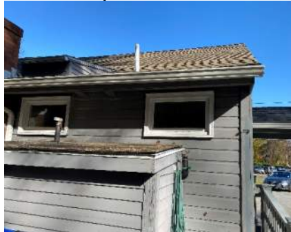
Awning windows at Toilet Rooms
