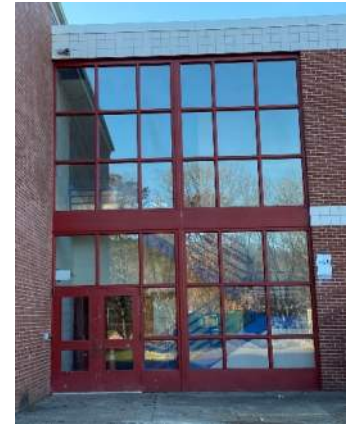
Curtain wall window at east entrance, rear
