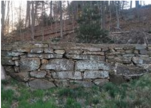
Stonework to resemble existing foundation in park
