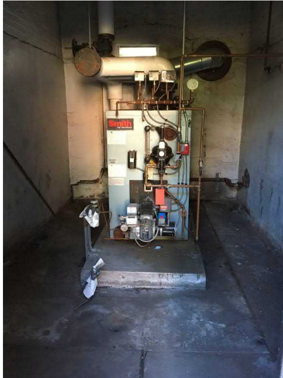
Furnace in Utility Room Extending From East End of Bld 81-106 (Note feed and return lines from Former USTs (REC-9) cut & capped, but remain in place)
