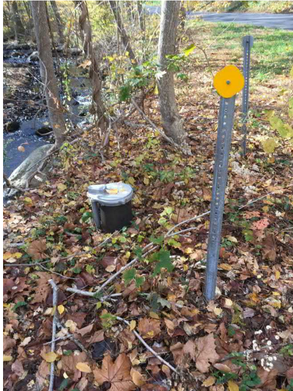
Water Supply Well With Water Line Extending to Bld. 81-115 Note Water Line to Water Pressure Tank in Bld. 81-115 Cut & Capped
