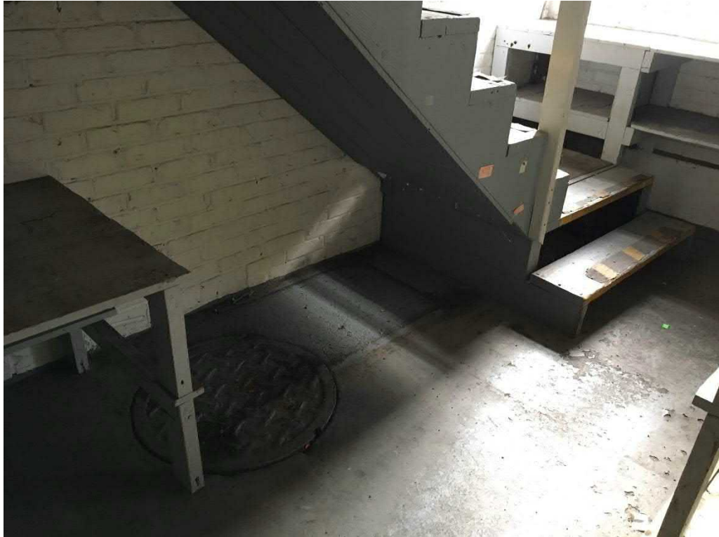
Manhole Access for Stormwater Line Extending Below Building 81-115
