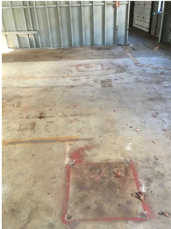
Markings of Former Above Ground Vehicle Lift At Building 81-106 (Note that this is a poured floor above a former below ground vehicle lift (REC 16))
