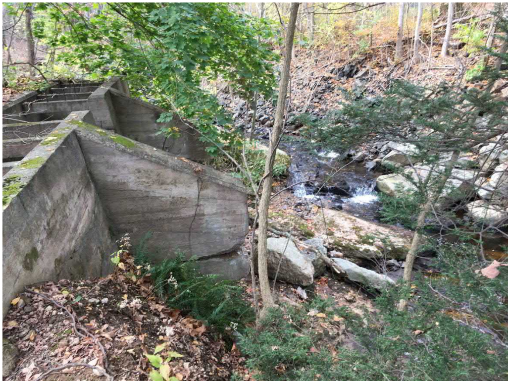
Former Flume Inlet with Remnants of Former Dam
