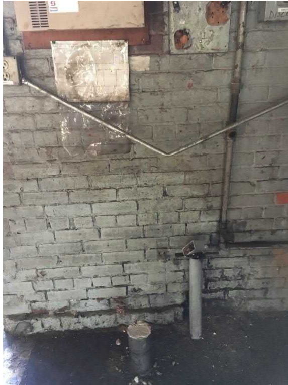
Waste Oil Drain Line to Former Waste Oil Tank (Rec-14) Bld 81-106
